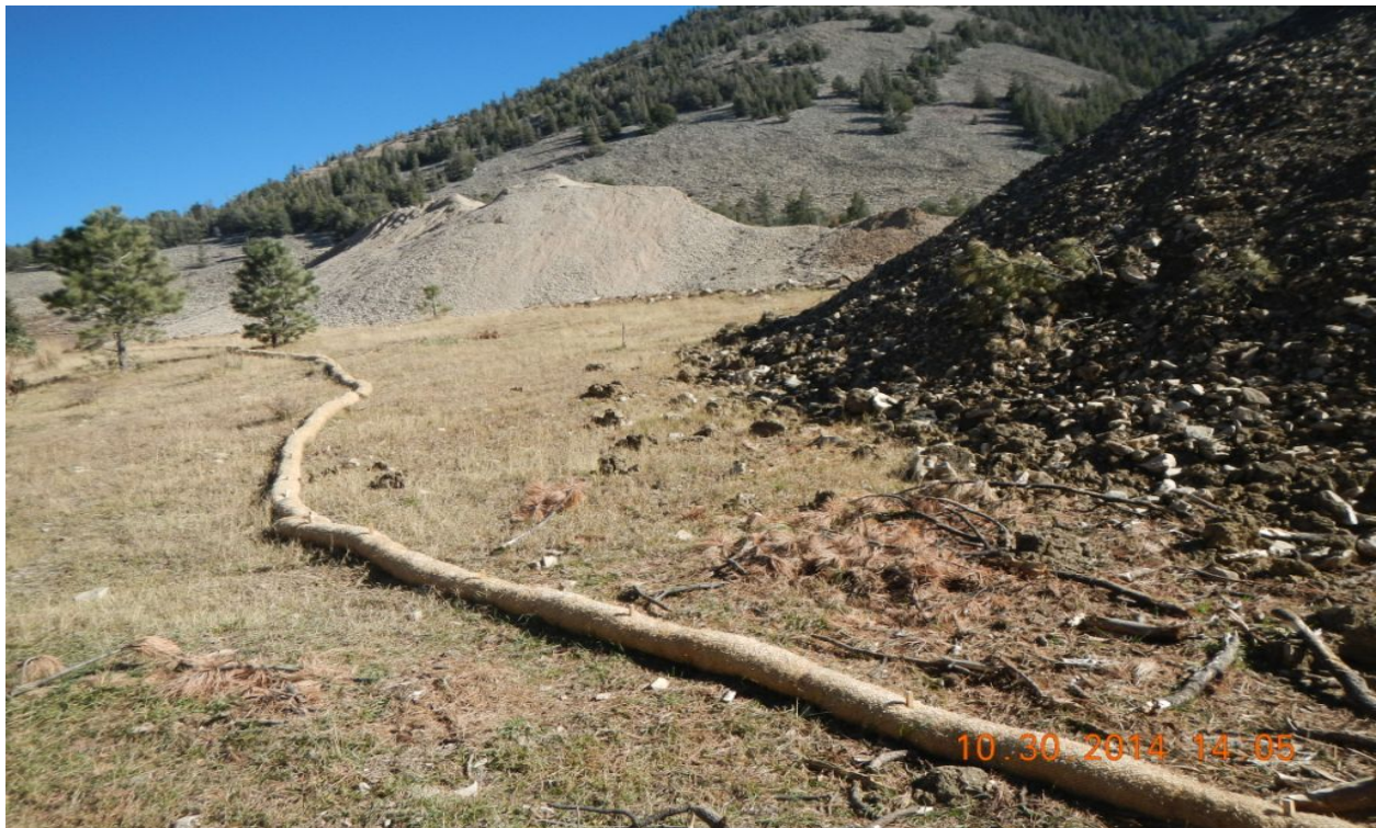
Erosion logs (8") around the pad and gravel pile
