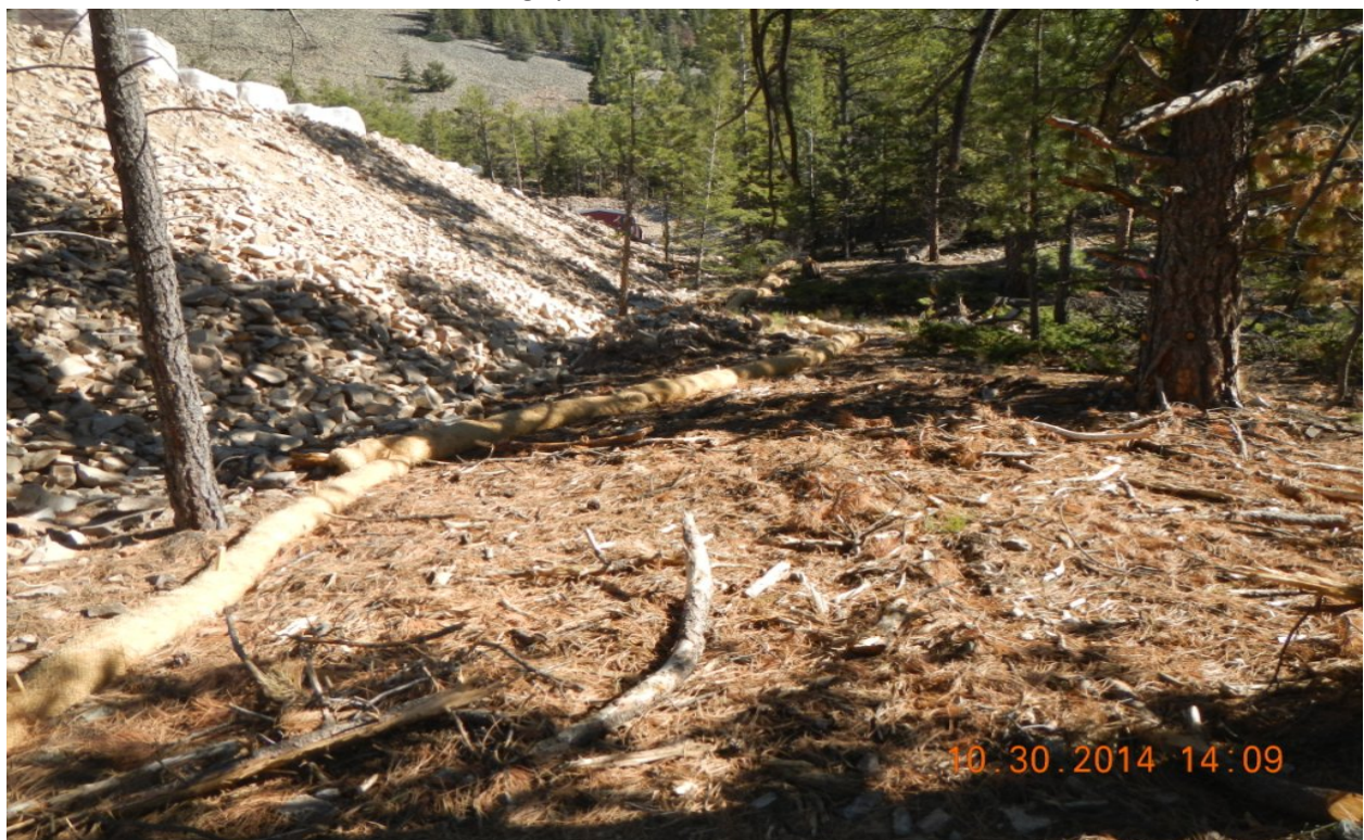
Southwest corner of location. Erosion logs placed around the downhill side of the location photo #6
