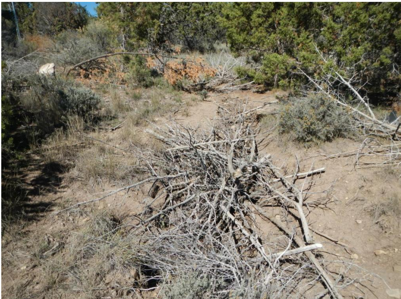
Photo 4. View of woody debris placed in erosional channel which will not likely be sufficient for stormwater control.
