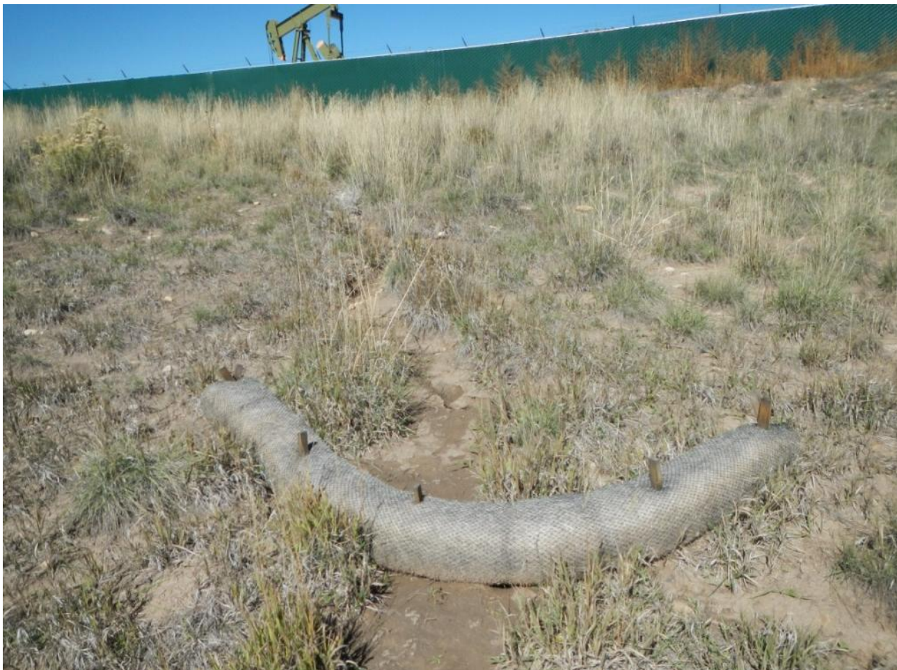
Photo 3. View of straw wattle that appears to be functioning within southern portion of project area.
