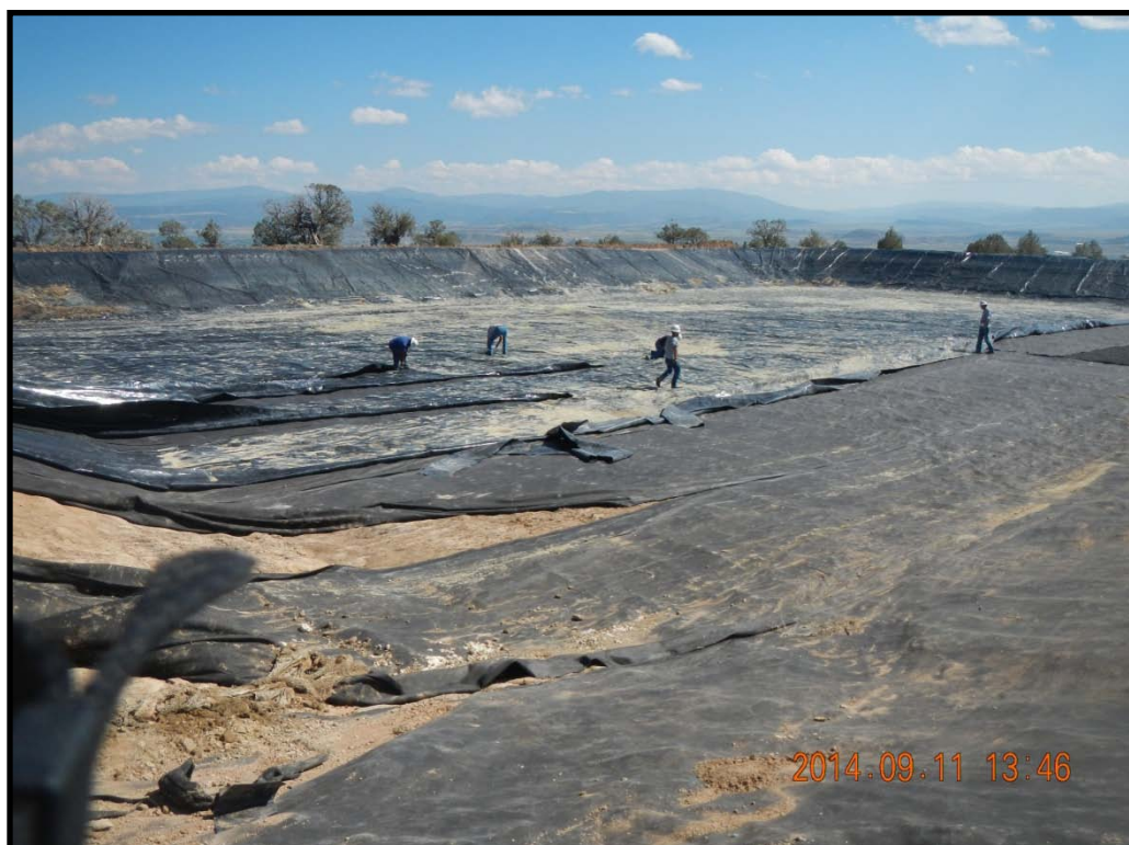
Removing the felt and the plastic portion of the liner.
