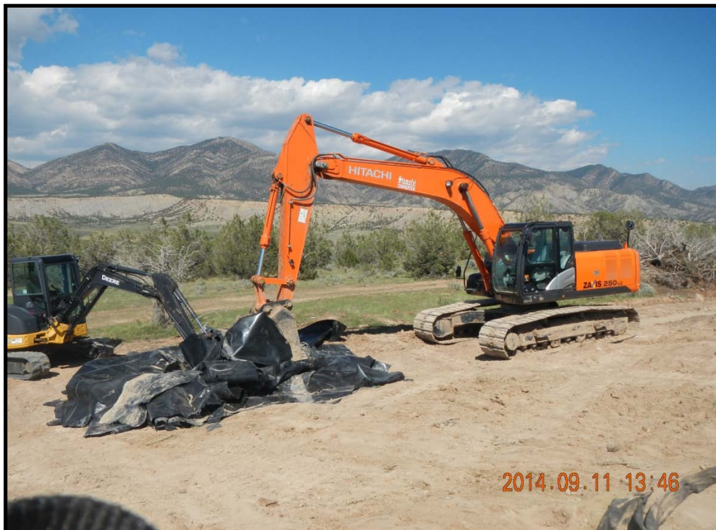
Wrapping up the plastic part of the liner for recycling (cut in 8' by 8' pieces).
