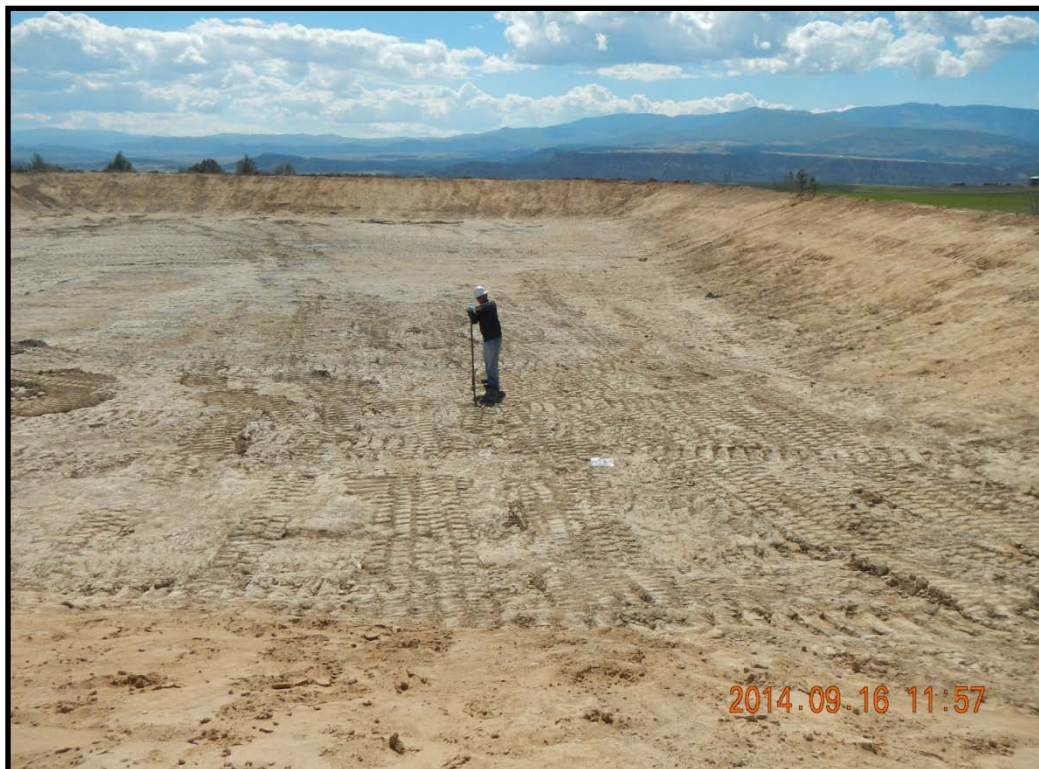
Pit liner removed. Consultant taking samples from the bottom of the pit.
