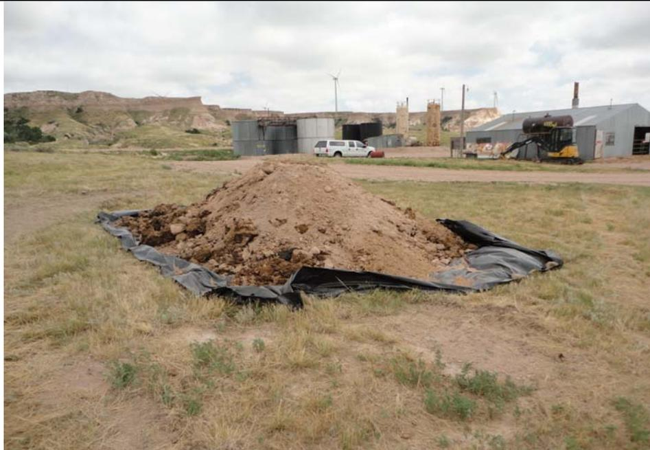
**Subject:** Impacted soils and E&P tank bottoms oily wastes were stockpiled on plastic. Approximately 10 cubic yards of impacted materials were estimated to have been removed.
