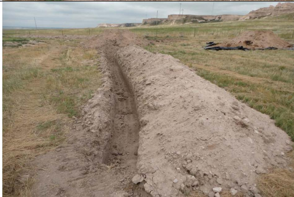
**Subject:** A trench was excavated around the perimeter of the south produced water pit, oily waste excavation. Impacted soils and E&P waste removed from the excavation were placed on plastic.
