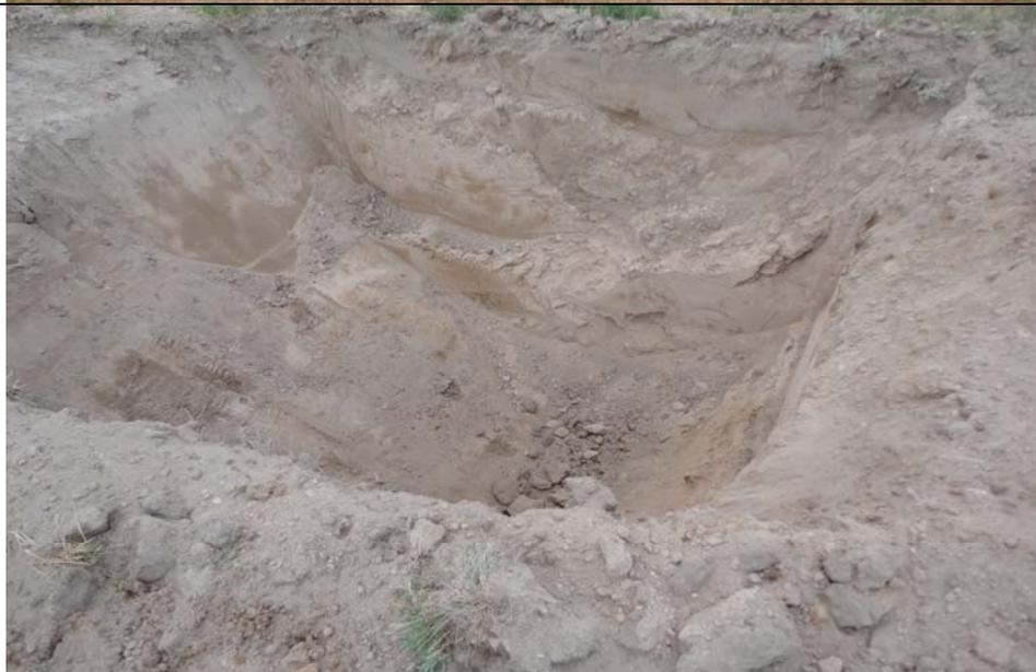
**Subject:** Photograph shows the excavation for the tank bottom wastes. The excavation measured approximately 10 feet wide by 15 feet in length and was approximately 8 feet deep.
