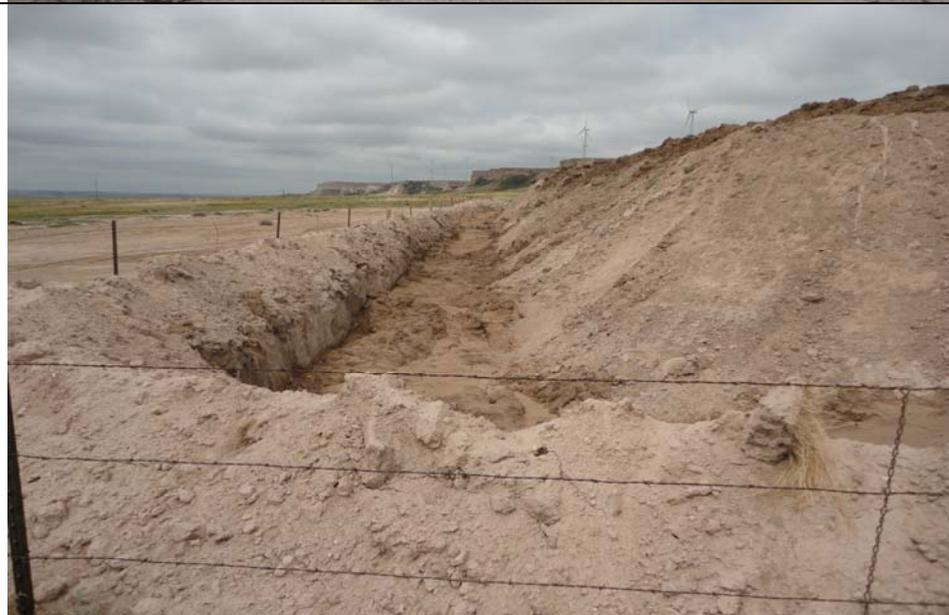
**Subject:** A trench and berm were constructed along the perimeter of the south pit to contain produced water during the repairs to the south berm.
