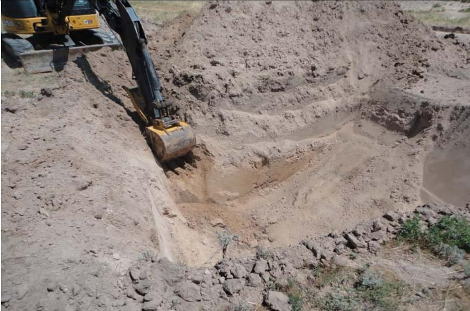
**Subject:** The excavator was used to collect soil samples from the side walls and base of the tank bottom waste excavation.
