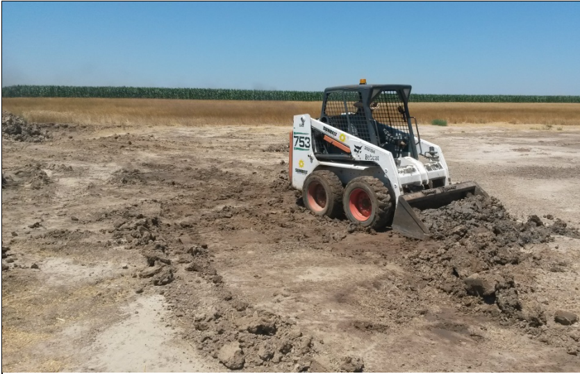
Photo 1 – Surficial removal of visually impacted soil on July 22, 2014
