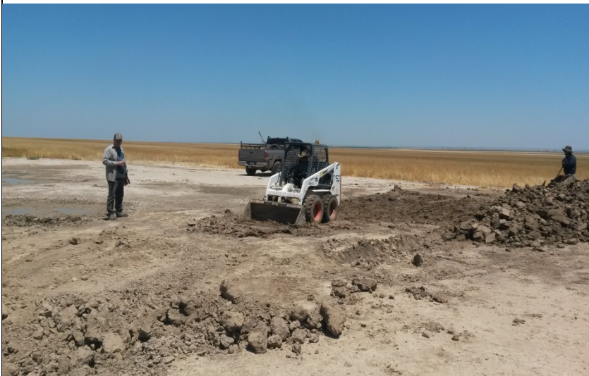
Photo 3 – Surficial removal of visually impacted soil on July 22, 2014
