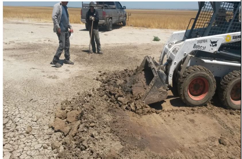
Photo 4 – Surficial removal of visually impacted soil on July 22, 2014
