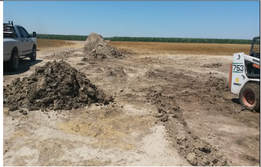
Photo 2 – Surficial removal and stockpile of visually impacted soil on July 22, 2014
