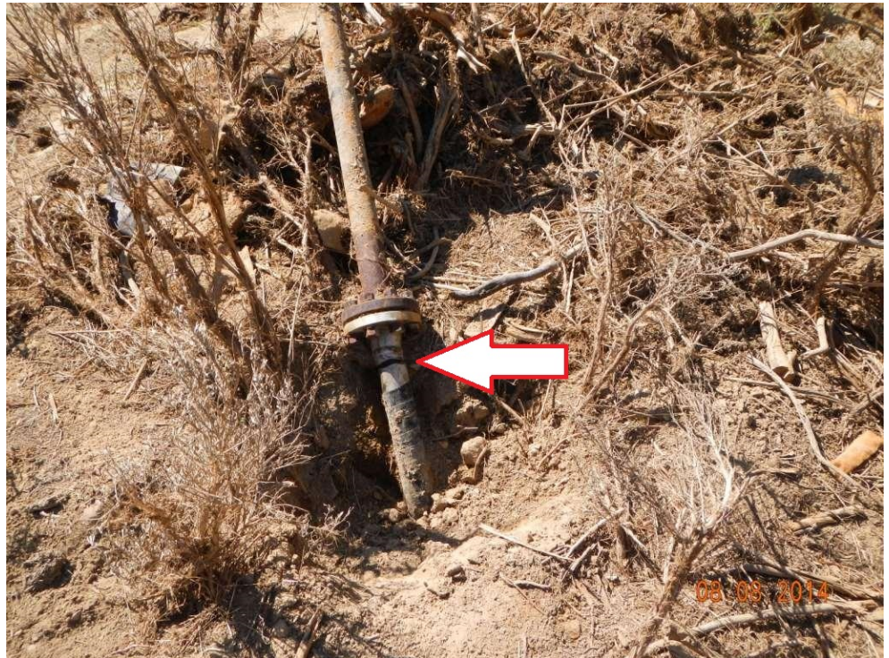
Damaged riser. Venting at time of inspection.
