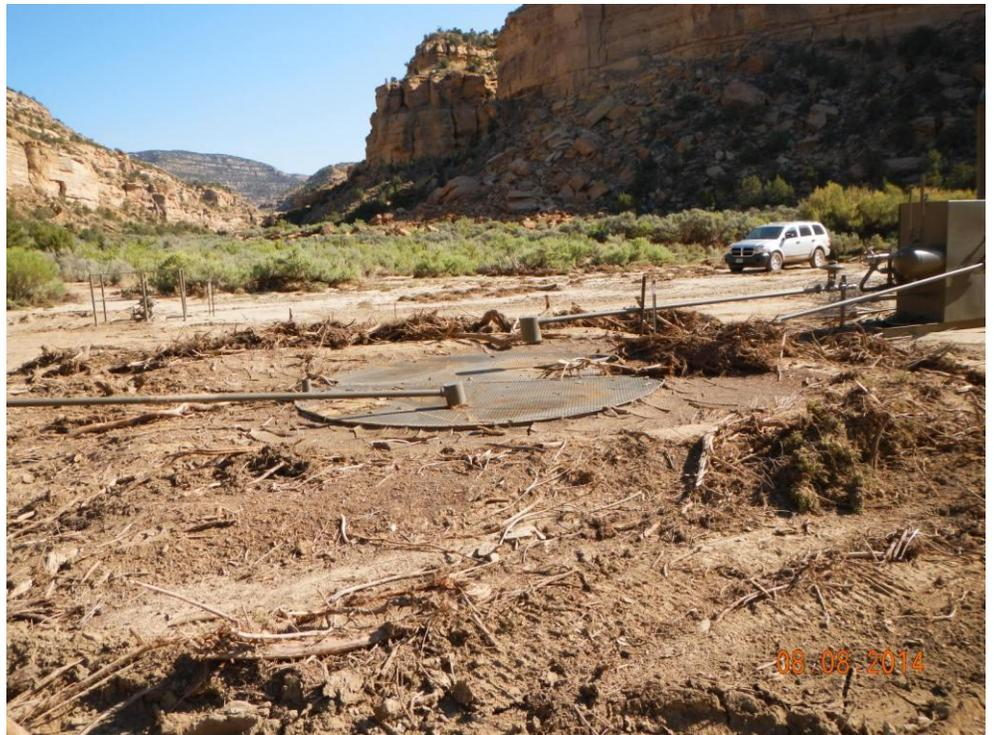
Blowdown tank at capacity w/ water still pumping into it at time of inspection.
