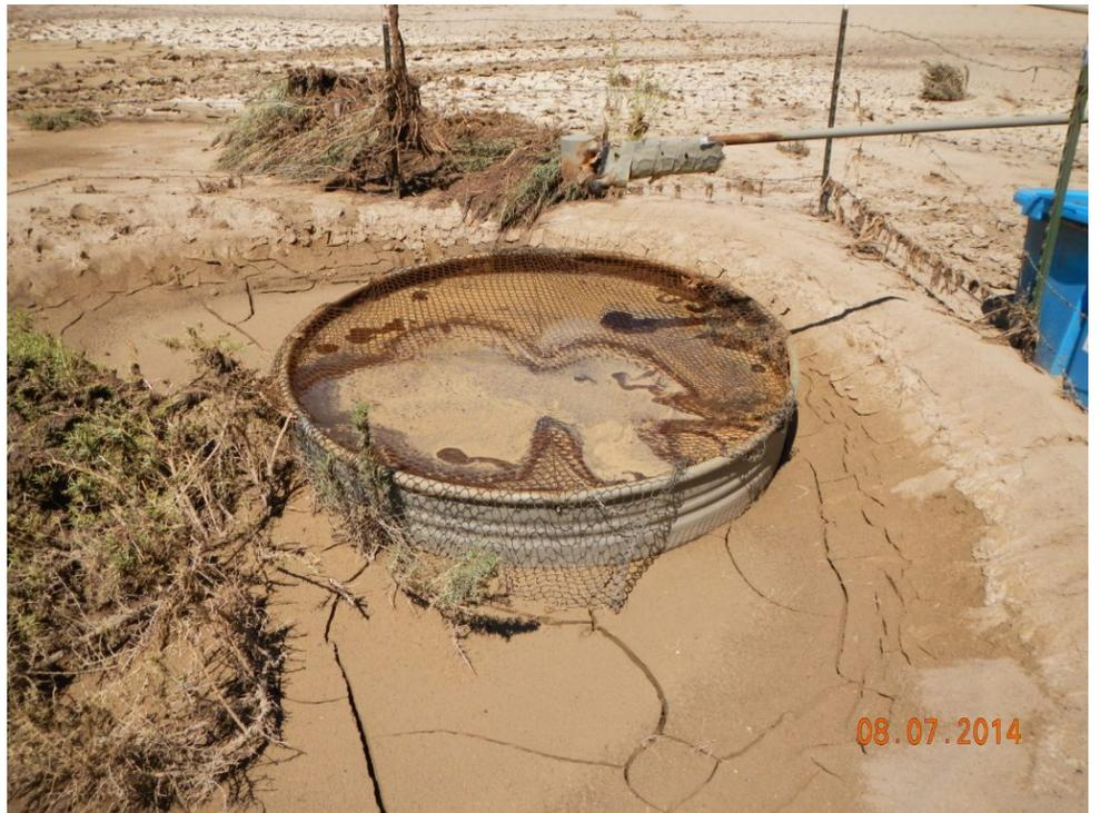
Meter run is leaning and appears to have been damaged by flood
