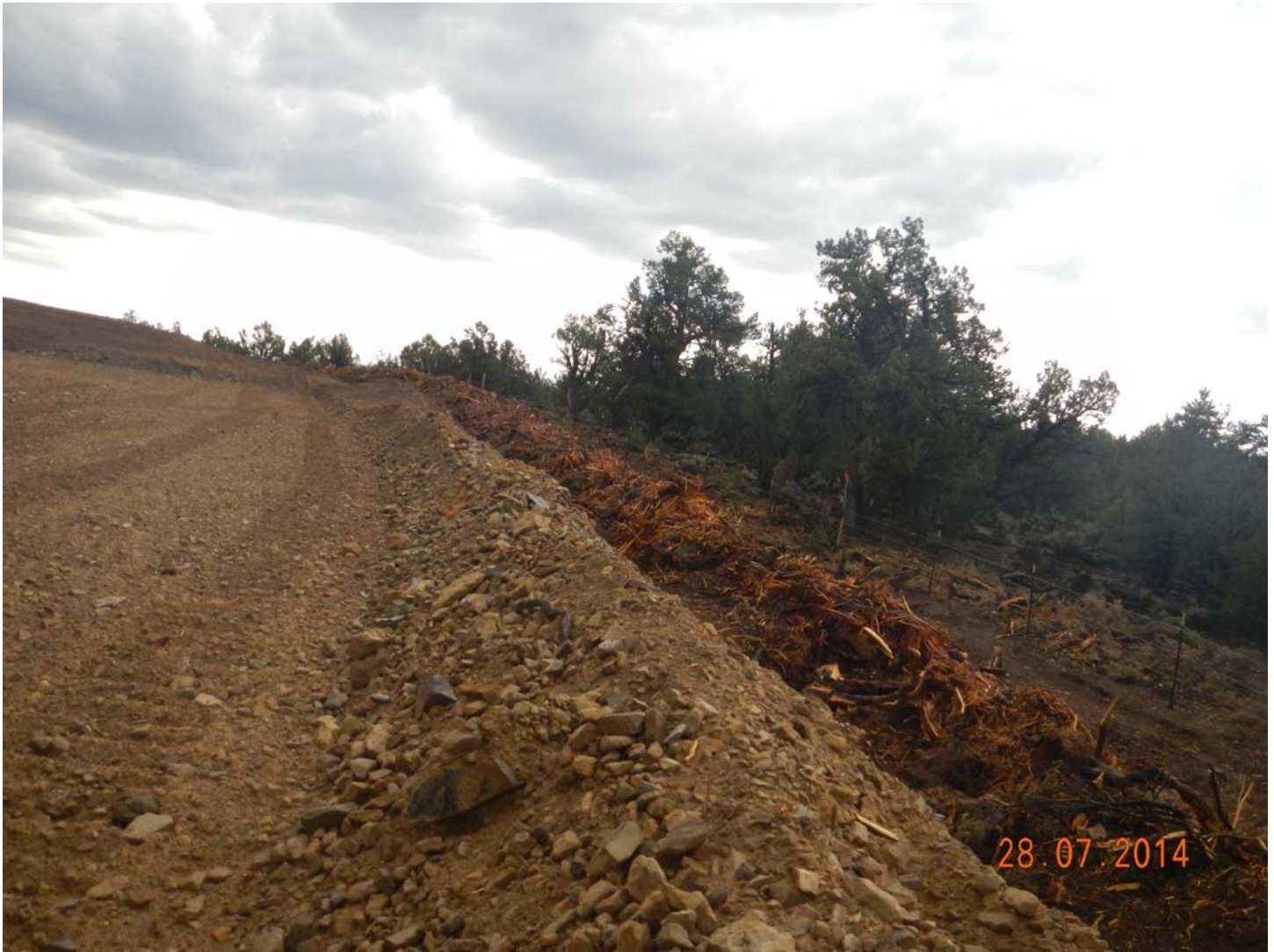
4.) Primary perimeter berm being constructed.
