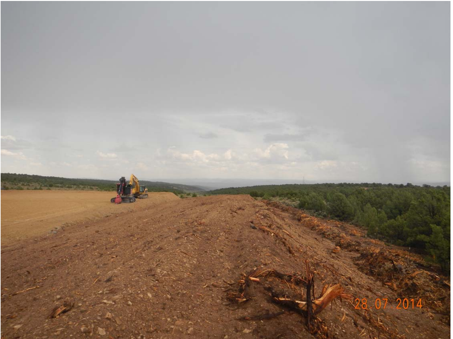
2.) Location stockpile being tracked. Slash utilized as BMP but contains a lot of topsoil without additional runoff BMPs.
