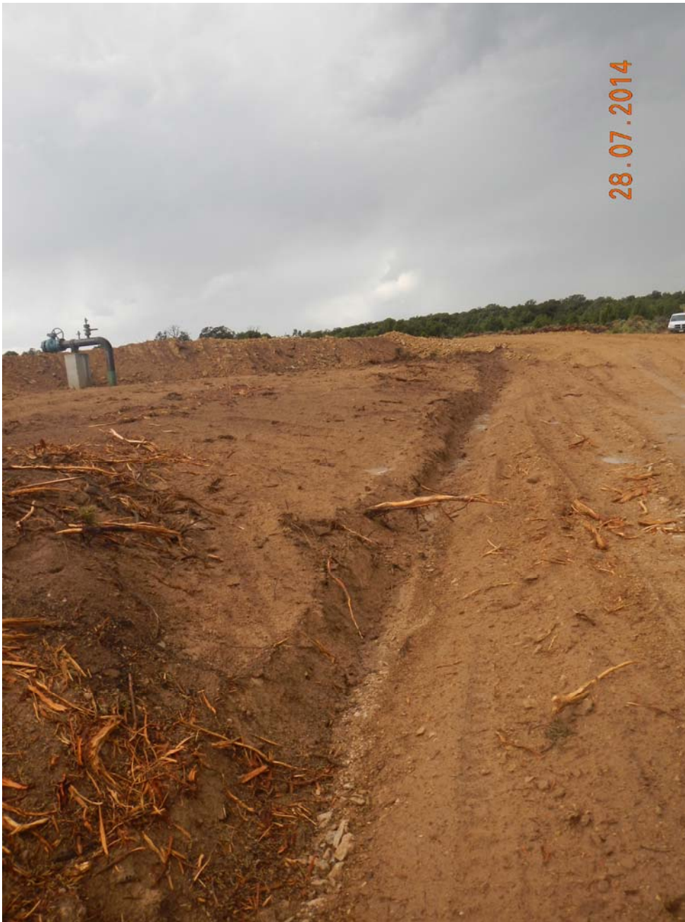
1.) Location entrance. Undercutting and sediment runoff observed.
