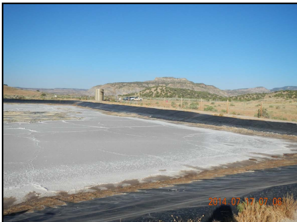
Dry pit. Sediments and salt cover most of the bottom of the pit. Bushes have been removed from around the pit but there is still some vegetation growing right on the border of the pit.
