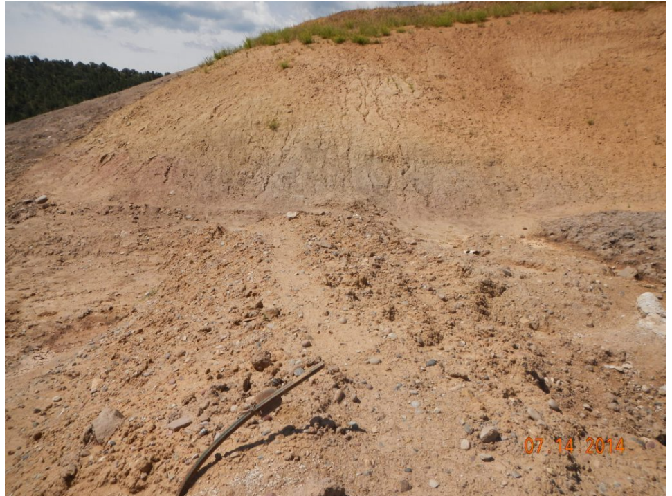
Erosion and rilling on cut slope. Trash in berm.
