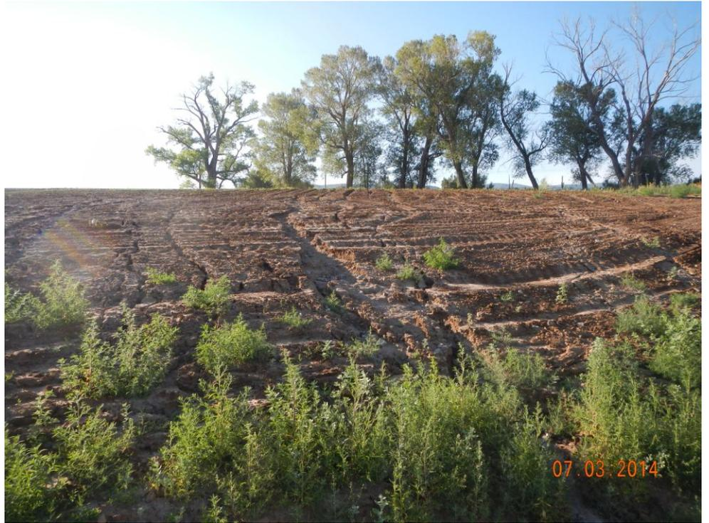
Some erosion and rilling on cut slope.
