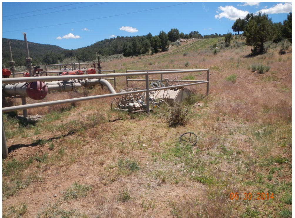
Valve parts and hand wheels stored at pig launcher.
