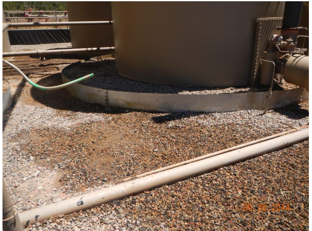
Staining around tank in containment.
