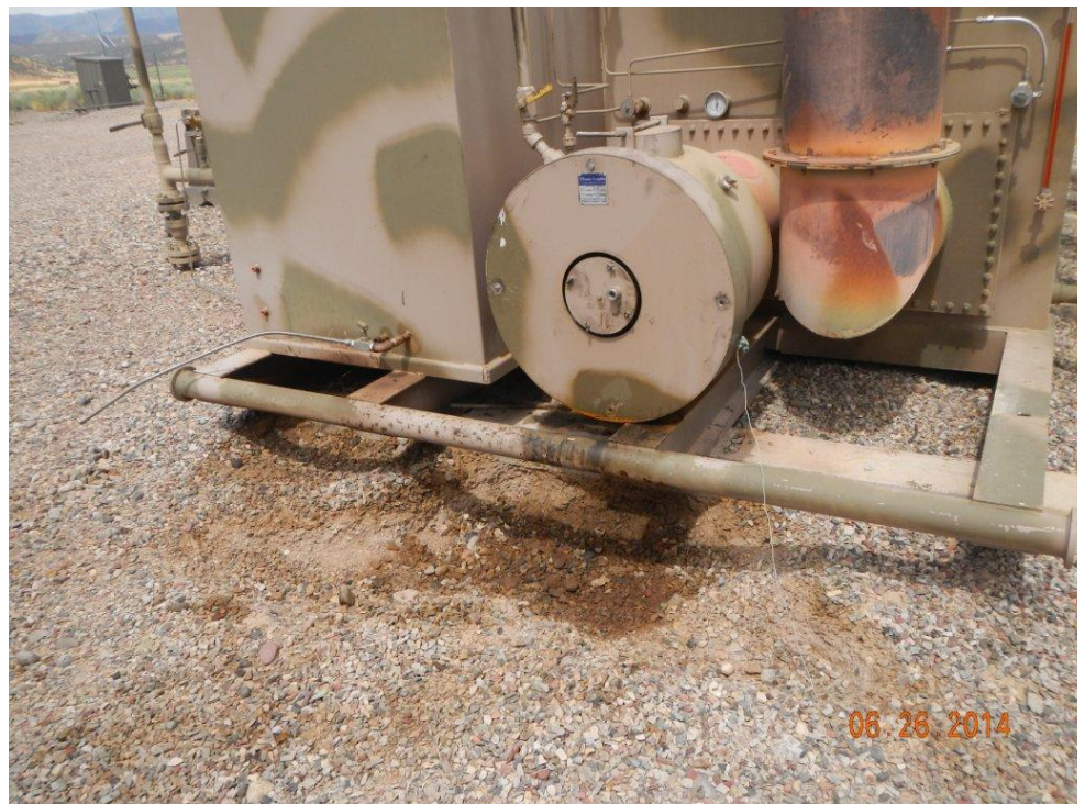
Staining at separators
