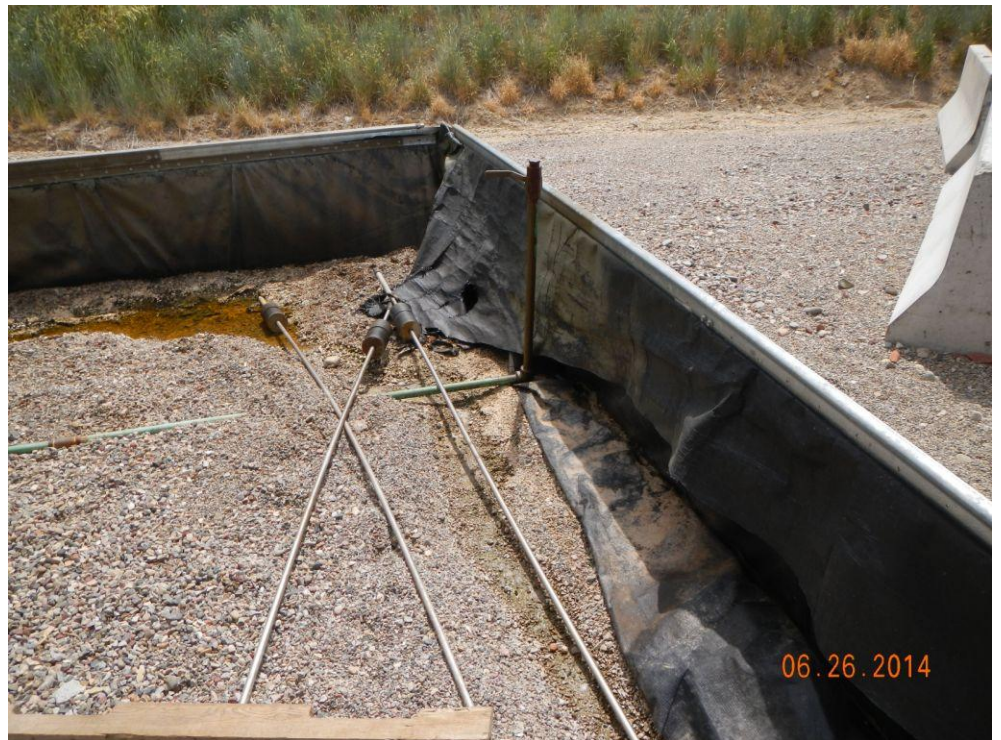
Damaged Containment
