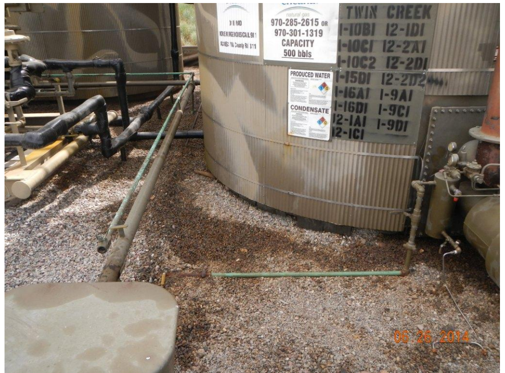
Staining in tank battery
