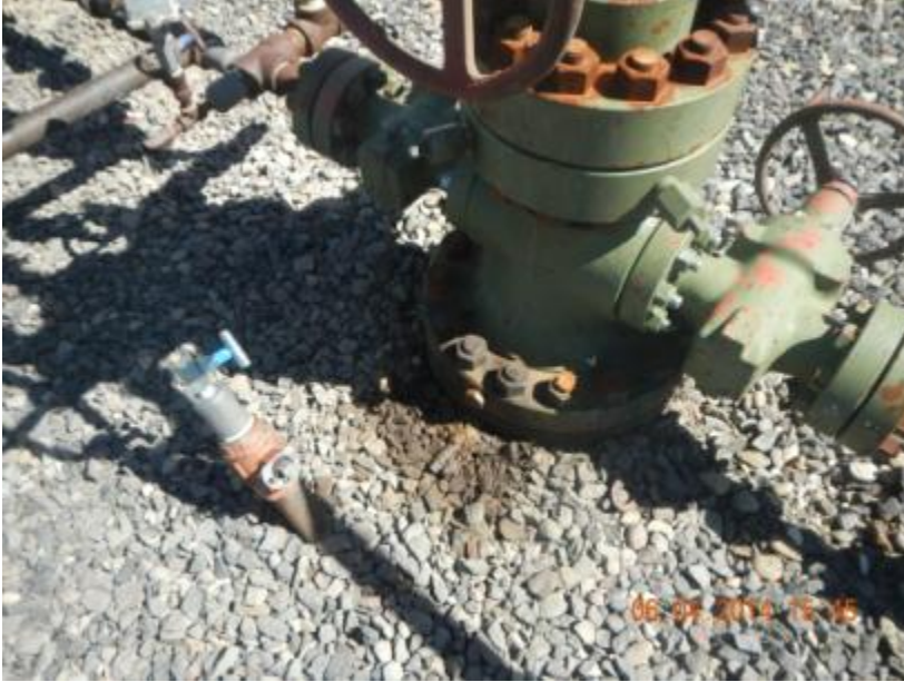
Staining from leaking around valve stem.
