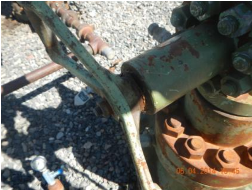
Leaking around valve stem
