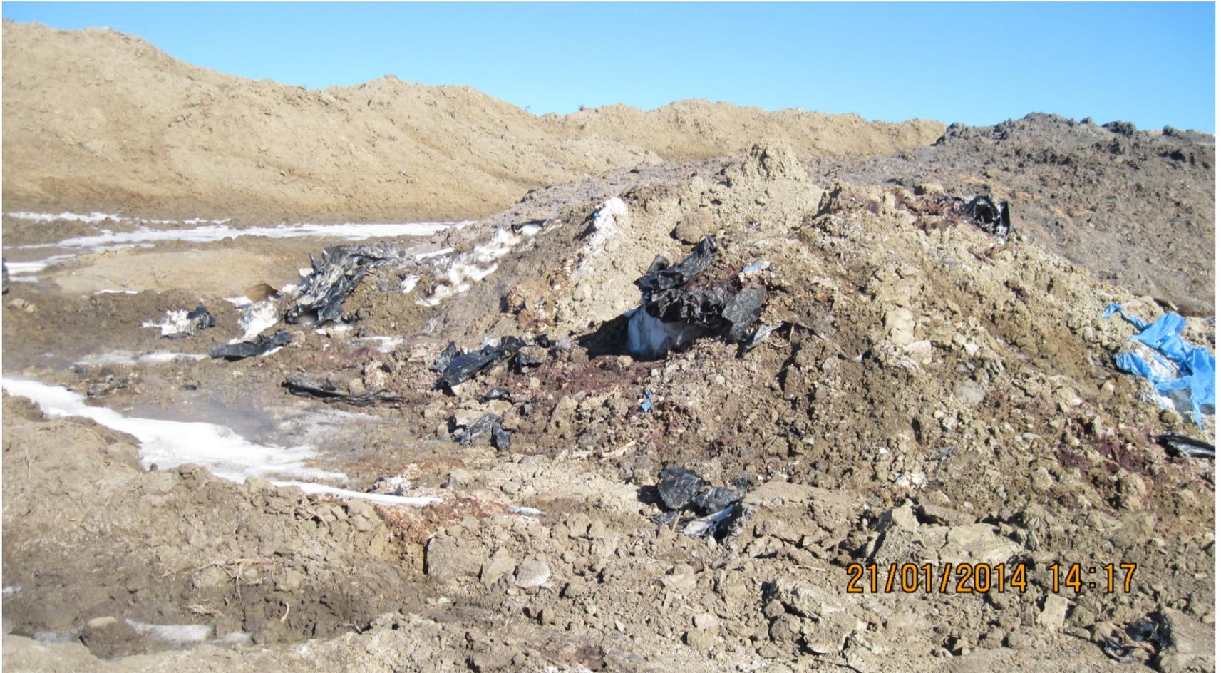
North side of location, no berm on E&P waste, trash blowing around location
