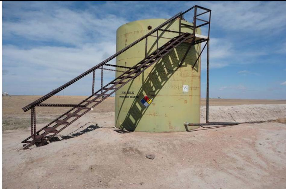
**Subject:** A 300-barrel capacity produced water tank was present on the northwest corner of the produced water pit, and was present in the 2009 Aerial Photograph showing the former skim pit.
