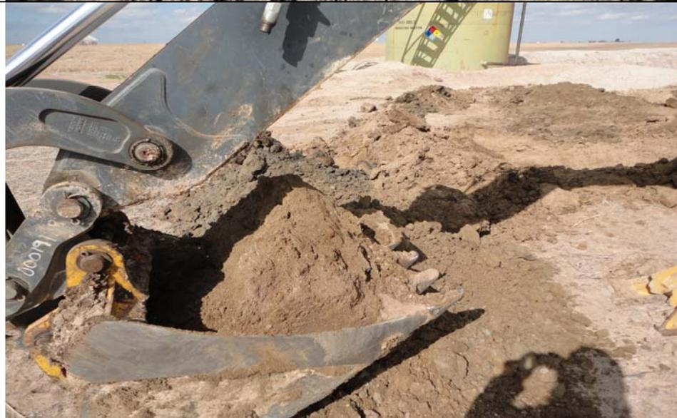
**Subject:** The vertical extent was defined in the west side wall trench by excavating to approximately 8 feet bgs. Soils consisting of clayey silt did not exhibit staining or odor. The headspace PID reading was 20 ppm at 8 feet bgs.
