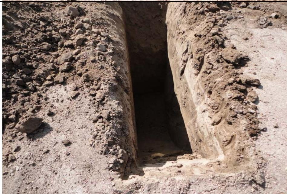
**Subject:** Impacted soils were not detected in the north trench skim pit side wall excavation at a depth of 8 feet bgs. The photoionization detector (PID) headspace reading was 20 parts per million (ppm) at 8 feet, and was 204 ppm at 5 feet bgs.
