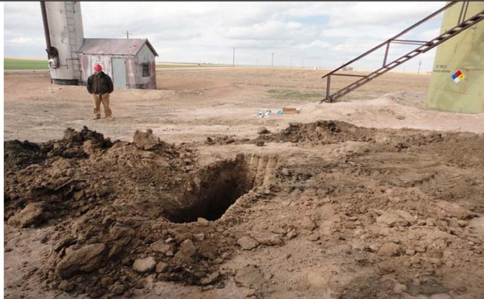
**Subject:** Impacted soils exhibiting staining and odor were detected in the west side wall trench excavated in the vicinity of the former skim pit. Impacted soils were encountered at approximately 4.5 feet bgs.
