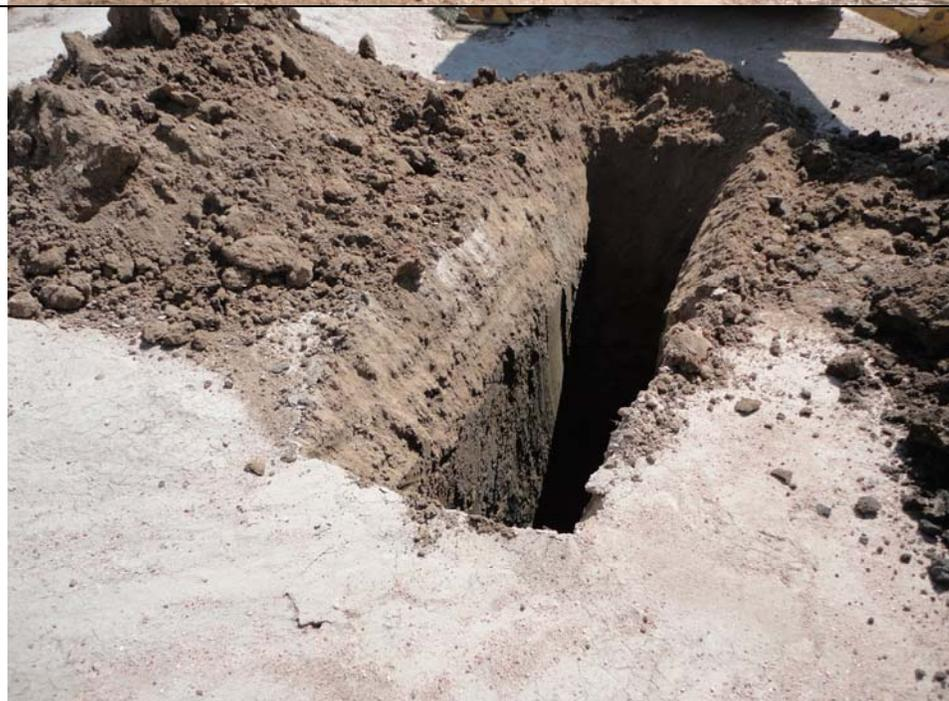
**Subject:** Impacted soils were encountered at approximately 2.5 feet below ground surface (bgs) in the trench on the east side of their former skim pit. The impacted soils had an odor and were observed to have black staining which extended to approximately 9 feet bgs.
