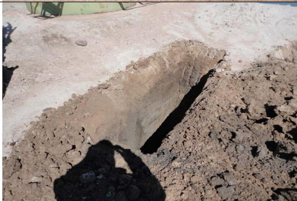
**Subject:** Photograph shows soil staining and the north side wall trench in the vicinity of the former skim pit. The photoionization detector (PID) headspace reading at 4.5 feet bgs was 94 parts per million (ppm), and the PID headspace reading at 8 feet was 154 ppm.
