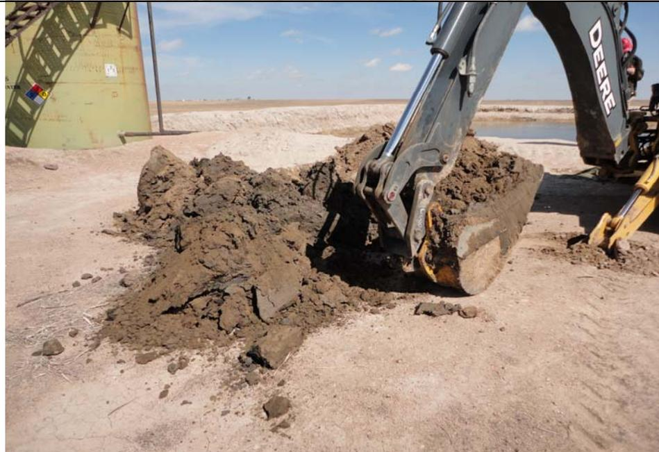
**Subject:** A north side wall trench was excavated in the area of the former skim pit location. Impacted soils were encountered at approximately 4.5 feet bgs.
