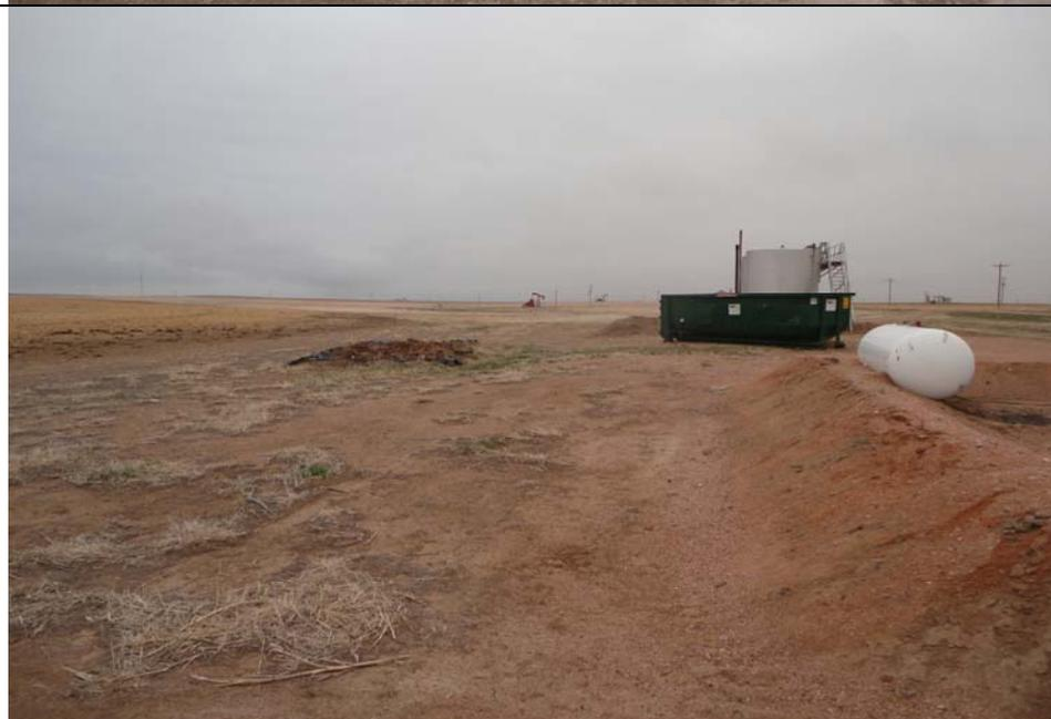
**Subject:** A Waste Management roll off dumpster was brought on location to haul off impacted soil from an April 2013 release from the vertical separator. The soil was stored on plastic and was loaded into the dumpster.
