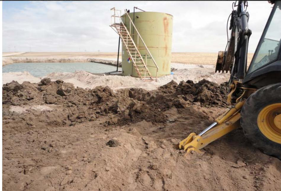
**Subject:** A north trench was excavated on the northeast side of the west pit area. Impacted soils were encountered at approximately 4 feet bgs. Excavated trench to a total depth of 11 feet bgs.
