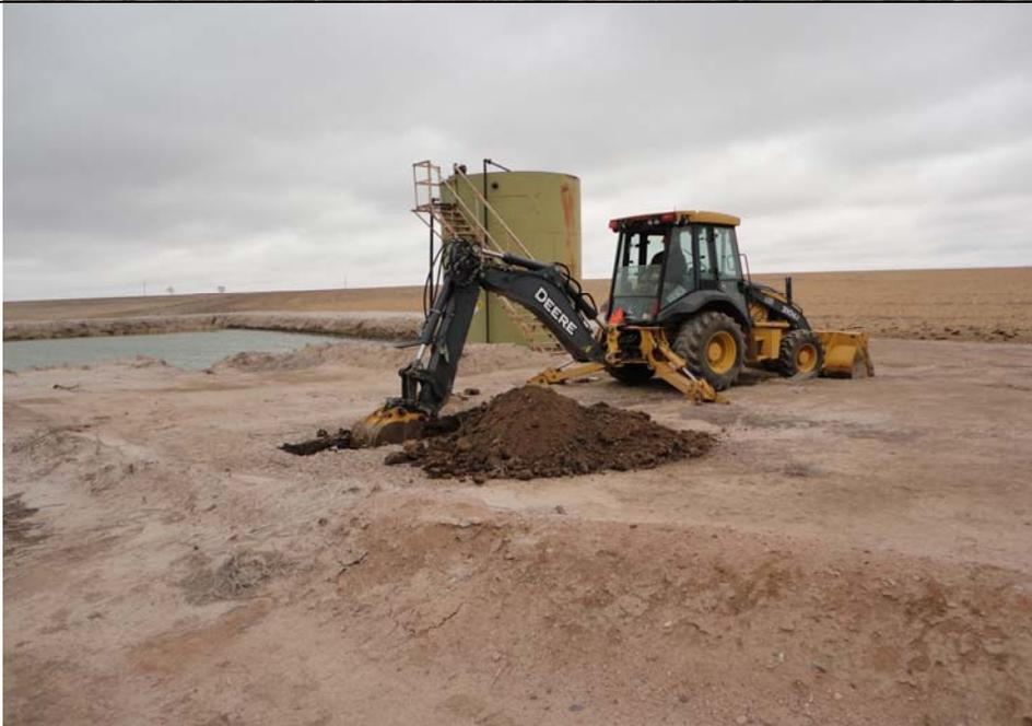
**Subject:** Assessment of the west pit began in a low area on the northwest corner of where the pit was shown in the 2009 aerial photo. Impacted soils were encountered at approximately 6 feet below ground surface (bgs). A partial earthen berm was observed on the west side of the former pit area.
