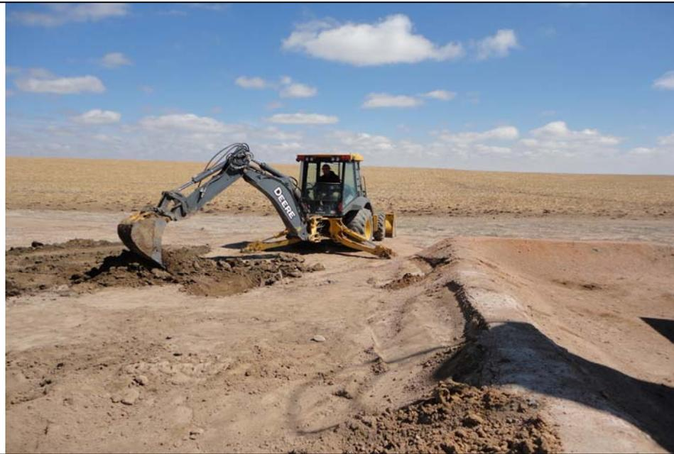
**Subject:** A trench was excavated on the southeast corner of the east pit. Impacted soils were encountered in the excavation. Photograph shows the location of the east trench in relation to the earthen berm for the vertical separator.
