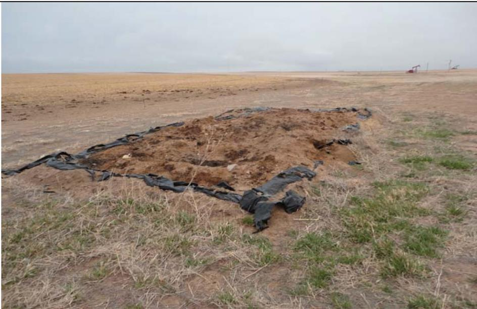
**Subject:** Photograph shows the soil stockpile from the vertical separator spill. The soil stockpile was loaded into the dumpster and was subsequently hauled offsite.
