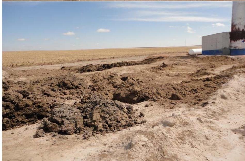
**Subject:** A buried produced water line was reportedly located on the east side of the stairs of the 300-barrel produced water tank and connected the tank to the vertical separator. A trench was not advanced in this area due to the presence of the line. Photograph shows an overview of the former east skim pit area.
