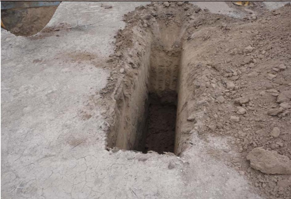
**Subject:** The southwest trench in the west pit area was advanced to a total depth of 8 feet bgs. No E&P waste or impacted soils were encountered in the trench.
