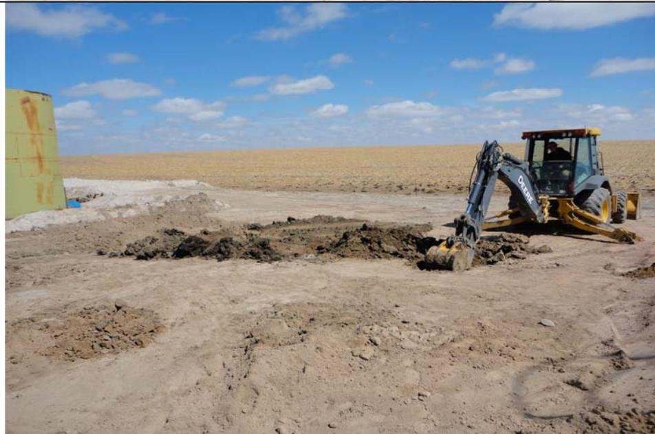
**Subject:** A trench was excavated on the east side of the east pit. Impacted soil and E&P waste was encountered at about 4.5 feet bgs.
