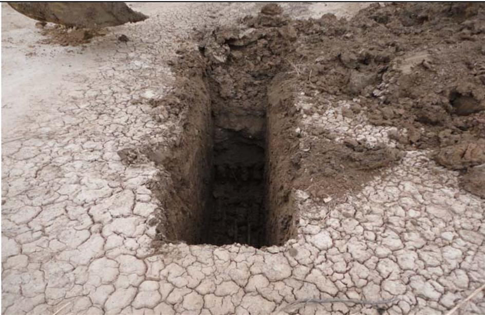
**Subject:** Shallow soils in the northwest trench were not impacted. Impacted soils were encountered at approximately six feet bgs. Soil sample CMOW-WP @ 6NW was collected in this area. Olsson directed the excavation to be advanced to ten feet bgs to define the vertical extent of impacts, and collected CMOW-WP @ 10NW.
