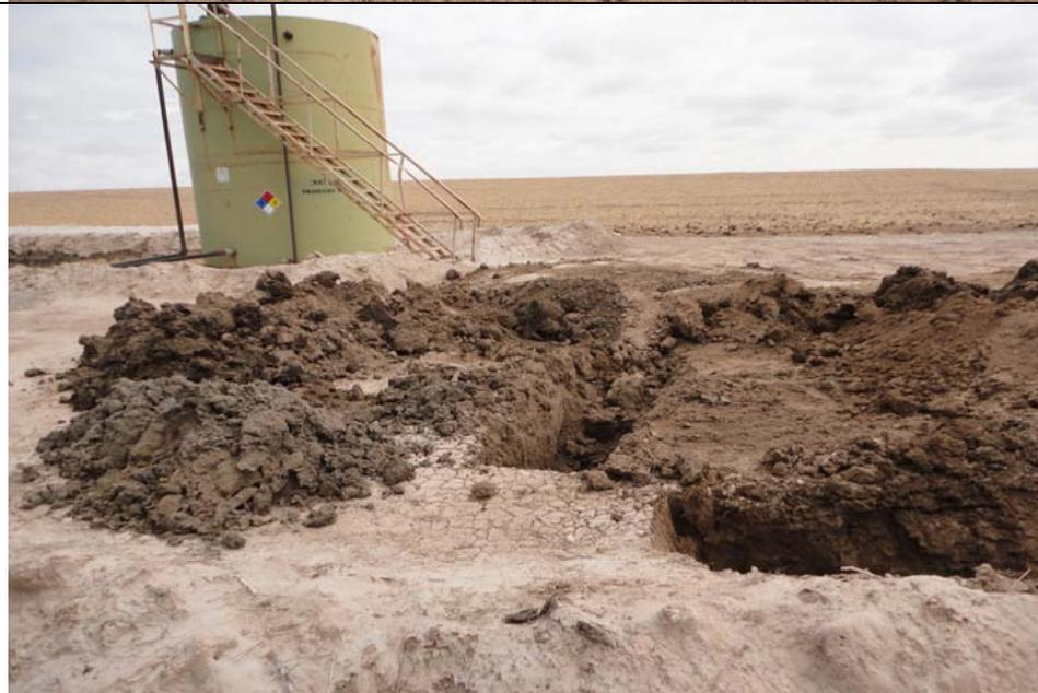
**Subject:** A trench was excavated on the west side of the west pit. Some impacted soils were encountered in the northern part of the trench at approximately 3 feet to 5 feet bgs. A soil sample CMOW-WP @ 7W was collected at 7 feet bgs and submitted for laboratory analysis.
