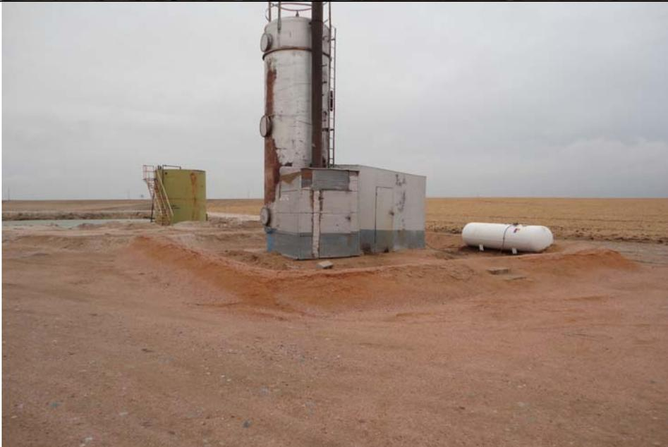
**Subject:** Oliver Warren #1 vertical separator and berm, 300-barrel produced water tank, and produced water pit. The location of the former skim pits is between the separator and the produced water tank.
