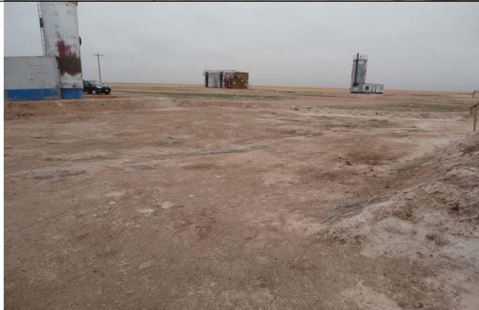
**Subject:** Photograph shows the location of the east skim pit at the Oliver Warren #1 site facing County Road YY and an adjoining separator and battery across the road to the west. A produced water line is reportedly present from the vertical separator in the upper left corner of the picture running to the 300-bbl produced water tank, and located to the right of the stairs shown on the right.
