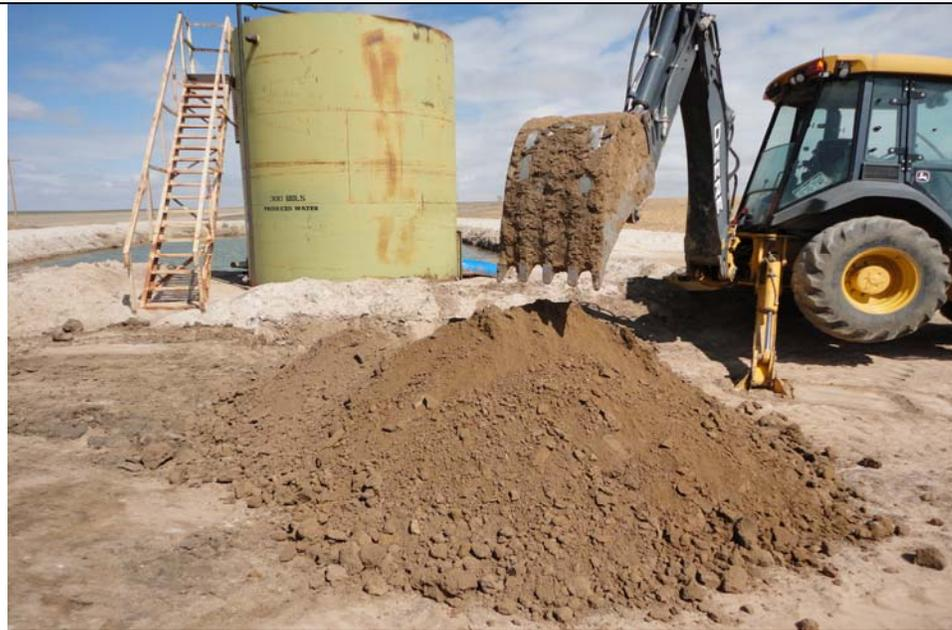
**Subject:** A trench was excavated on the north side of the east skim pit location near the produced water tank berm. Impacted soils were not encountered in the trench down to a total depth
