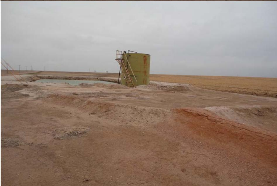
**Subject:** The location of the two skim pits at the Oliver Warren #1 site is shown in the partially bermed area in front of the 300-barrel produced water tank. Surrounding land use is agricultural and for oil production.
