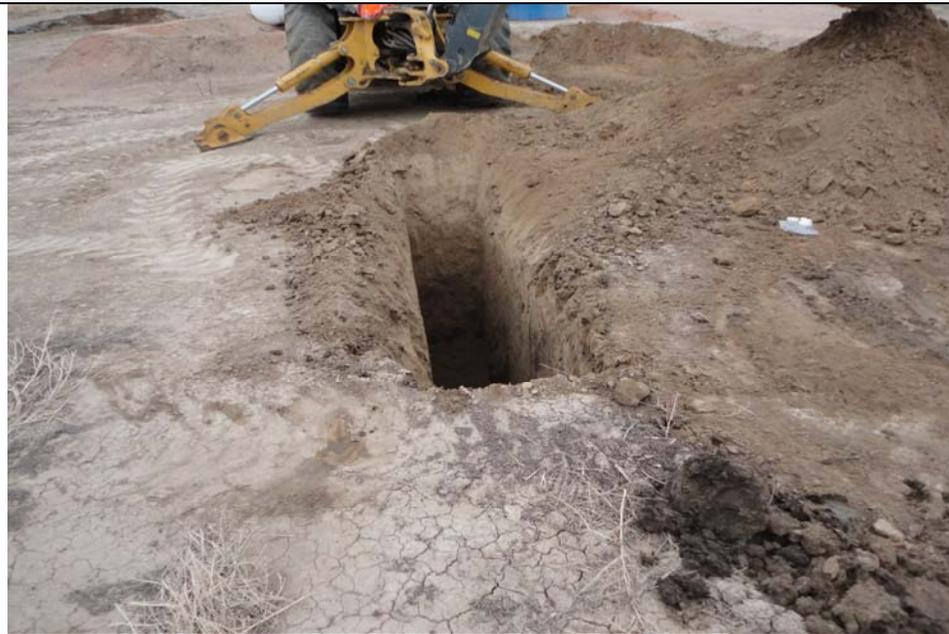
**Subject:** A trench excavated on the east side of the west pit did not show evidence of staining or impact. There was no odor or elevated PID readings recorded for soils down to nine feet bgs. A confirmation soil sample CMOW-WP @ 9E was collected.
