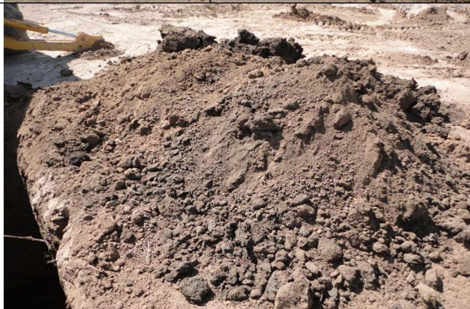
**Subject:** Impacted soil was encountered in the east trench of the east pit at approximately 4.5 feet bgs. Photograph shows excavated soils.
