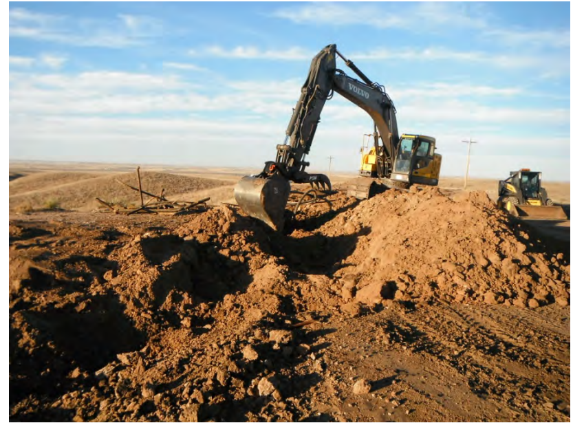
Excavation of impacted soils at tank battery location
