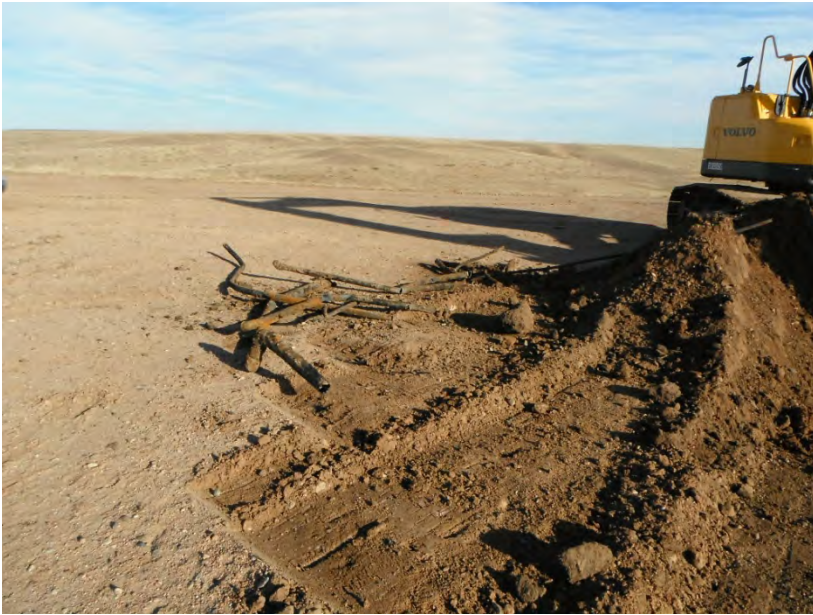
Removal of excess piping
