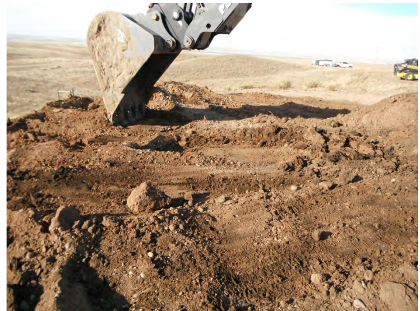
Excavation of impacted soils
