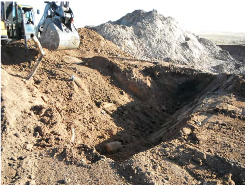
Excavation of impacted soils at treater location
