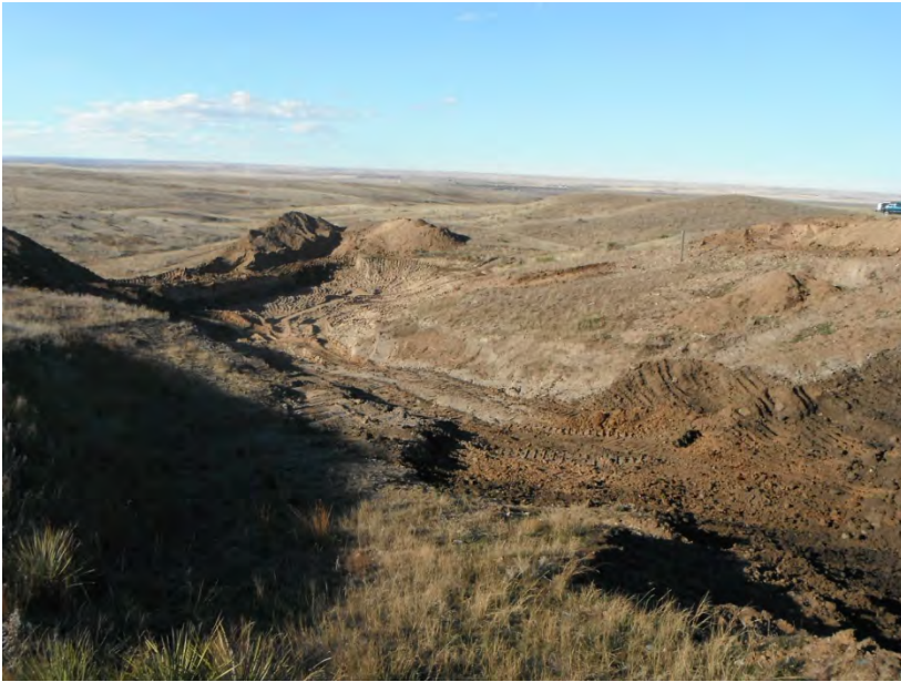
Pit area after impacted soil removal
