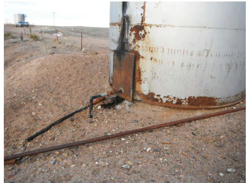
Undermined and rusted out tank above pits
