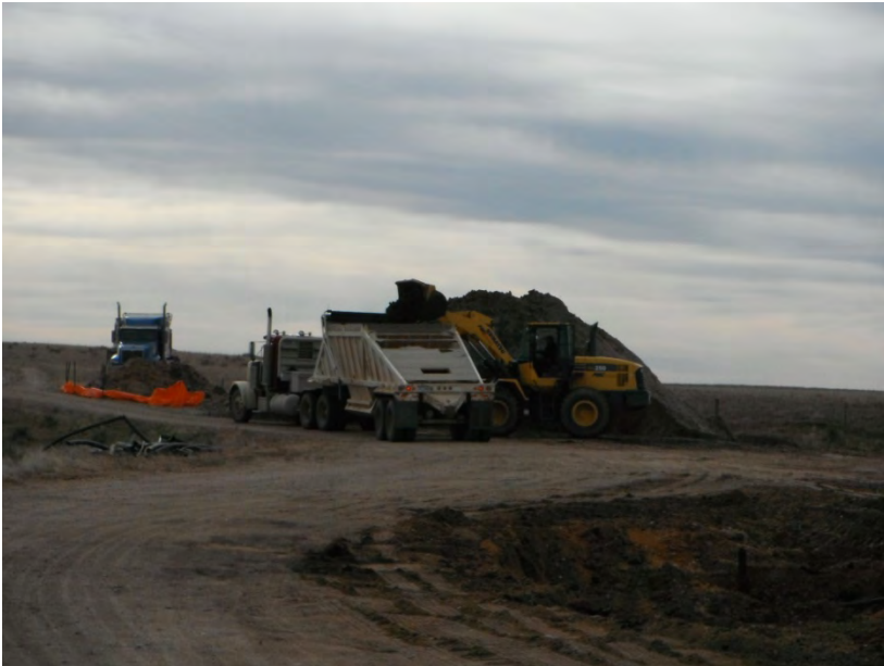
Loading out impacted soil to landfill
