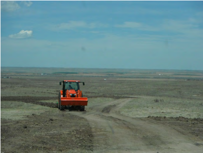
Ripping access road to relieve compaction
