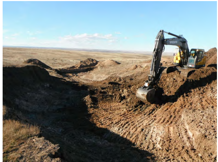
Excavation of impacted soils in upper pit
