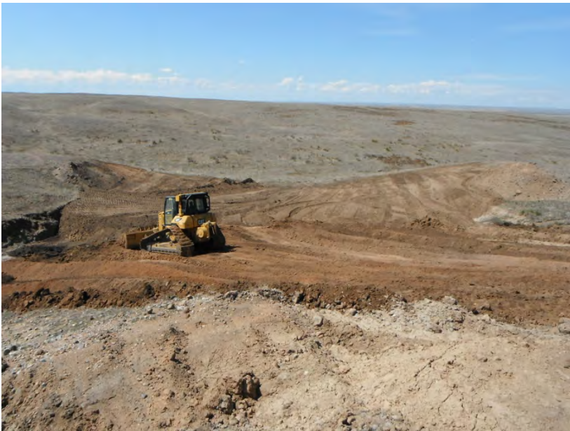
Regrading of pit area
