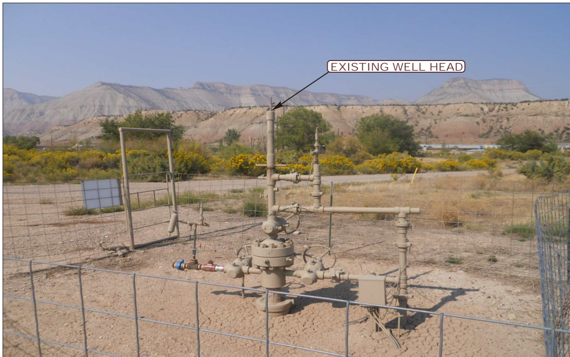
PHOTO: VIEW OF EXISTING WELL HEAD
