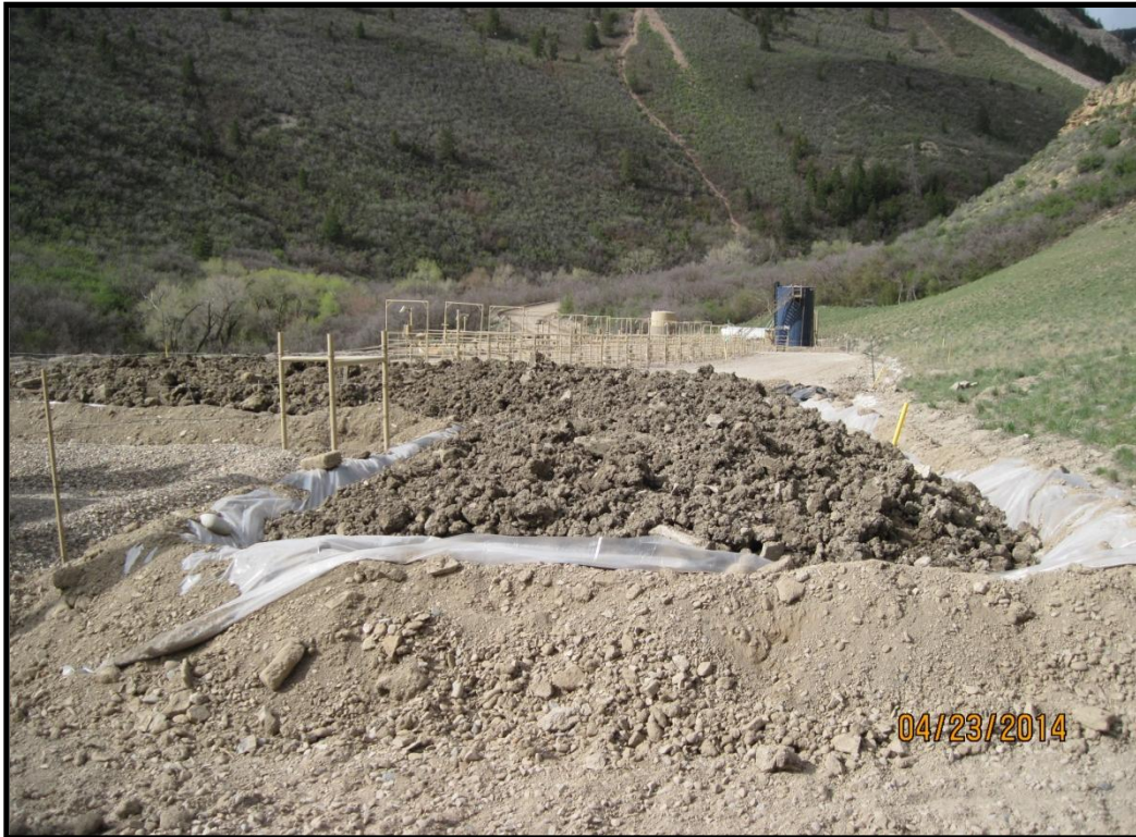
Temporary storage of material excavated during PBV removal.
