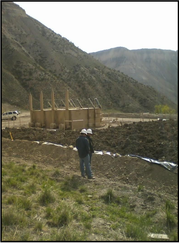
Material spread out in bermed area, about 3 to 4 feet thick for temporary storage.
