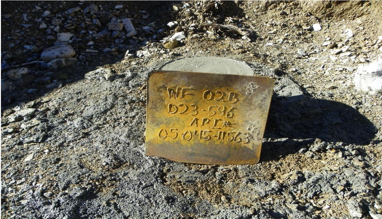
Cement was pumped to surface as shown. The metal plates were then welded atop each conductor.
