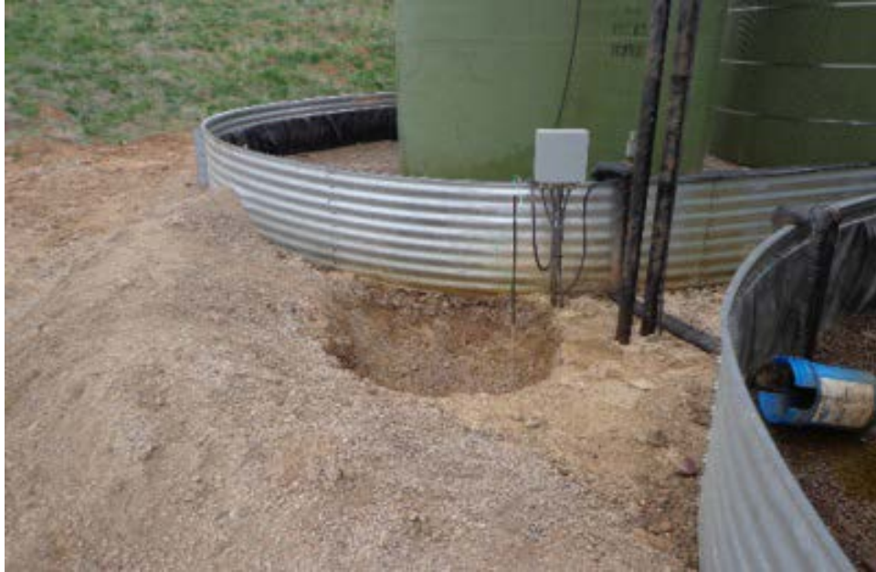
Photo 1 – Overspray excavation, approximate 5 foot radius by 2.5 feet deep.
