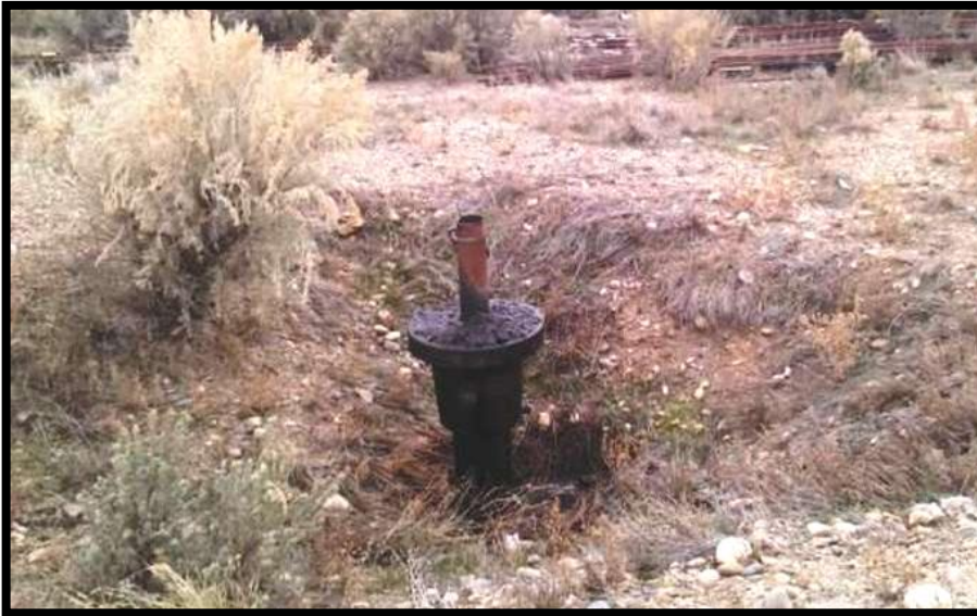
Exposed well casing and adjacent areas.
