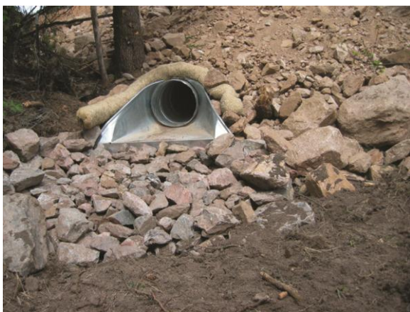
EROSION LOG CULVERT OUTLET PROTECTION
