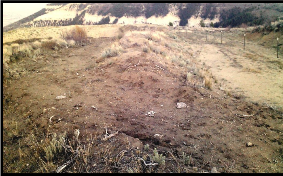
Viewing East along southern rim of well pad. Closure of road in process: Regrading, seeding, and fencing observed along this segment (to the right); and an interim access point created for further reclamation work, (center).
