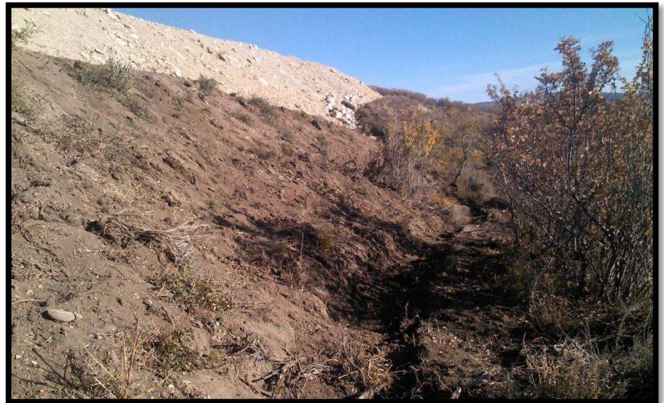
Double berming & ditches along fill slope sides.
