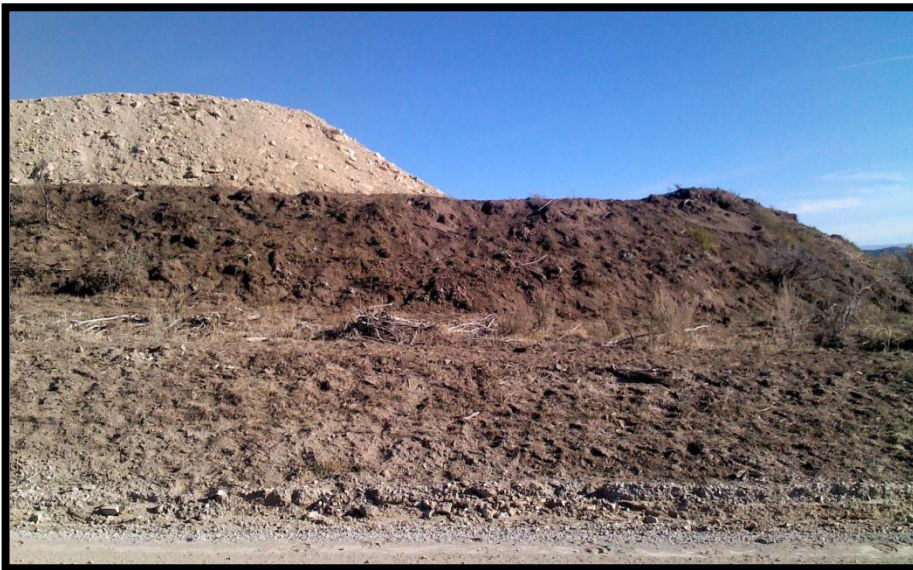
Stockpiled soils, secondary berming, and exterior slope of retention basin/sediment trap
