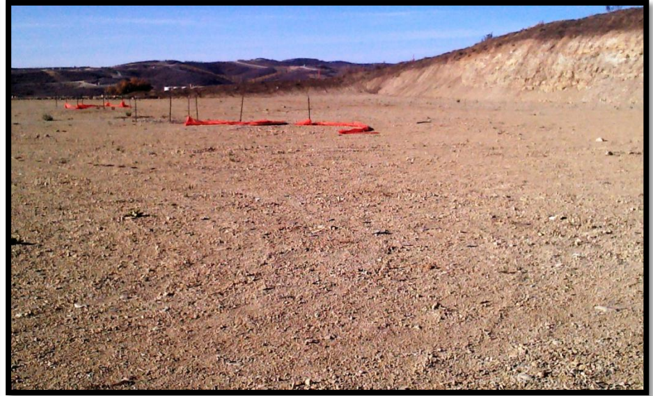
Viewing North: well pad footprint, markings for cellar/conductors, and stable cut slope.
