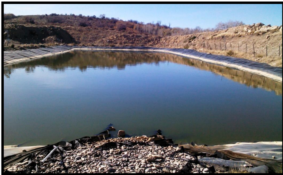
Viewing east, pit (CC Pond #3): Foreground: Surface protector ramp from hose intakes/outtakes.
