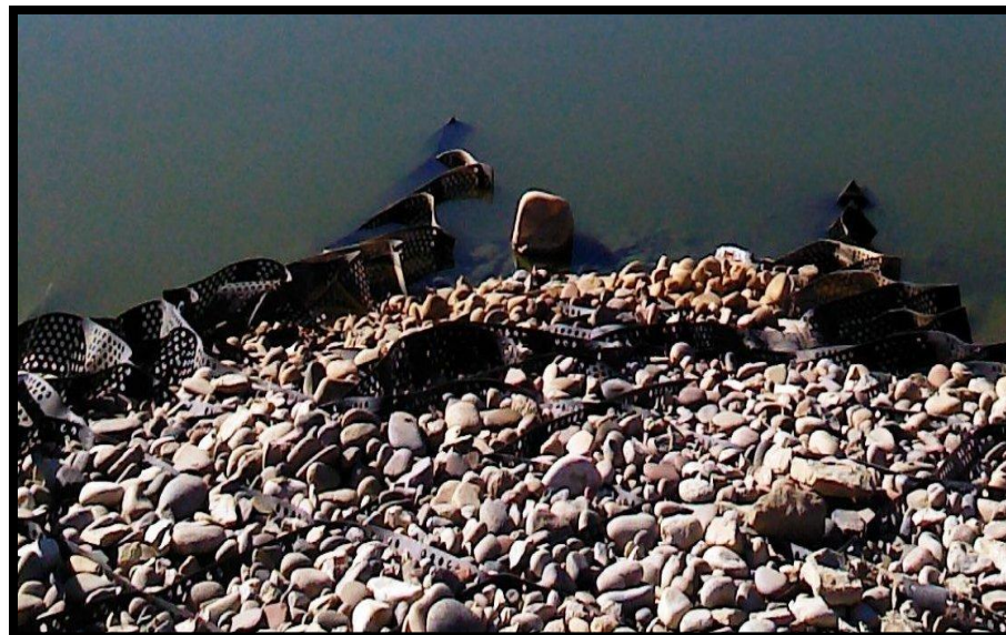
Close-up of surface protector ramp: Underlying plastic liner with cobble & plastic baffles.
