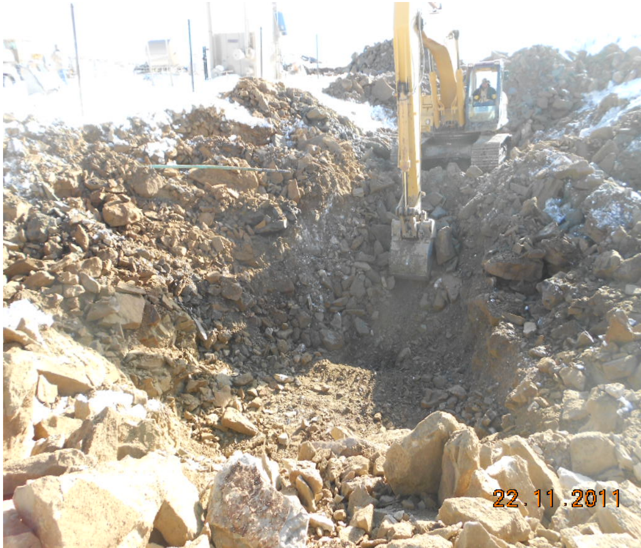
Visual representation of the impacted soils on pit bottom and pit walls during excavation
