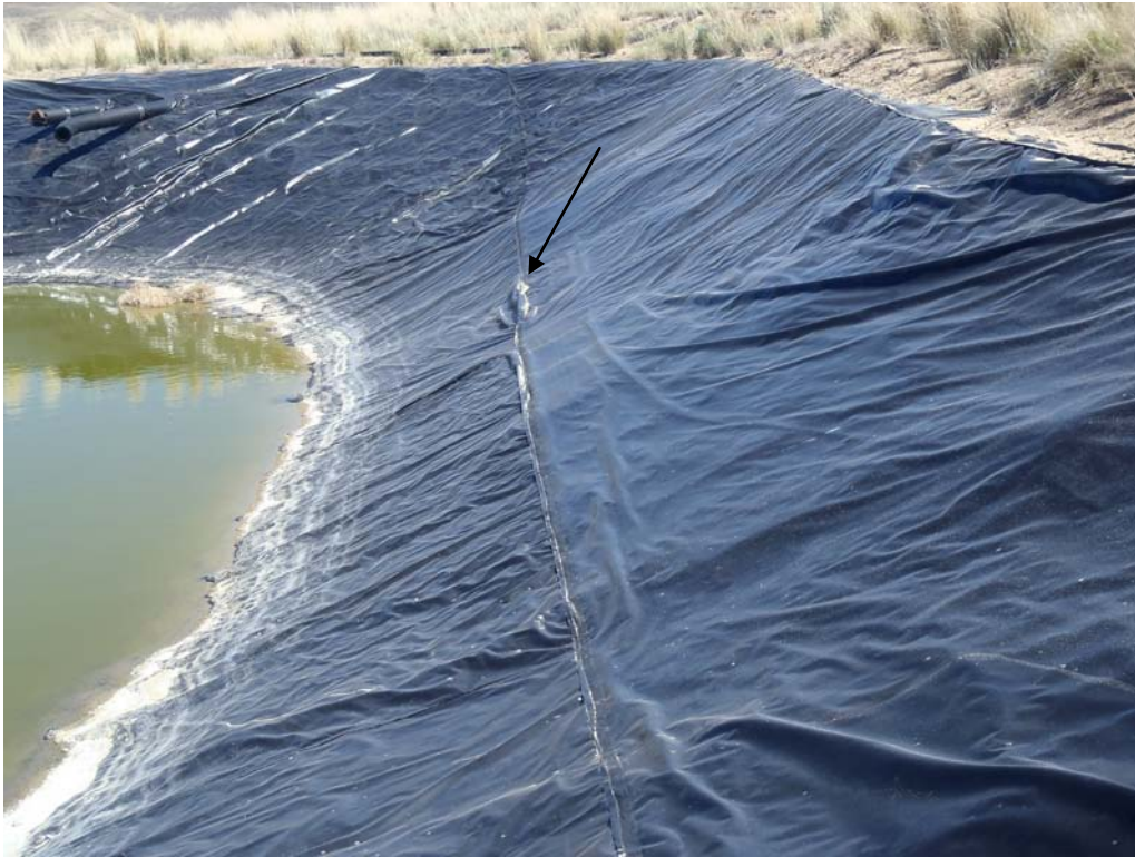
Xenon Lower Pit – Seam failure.
