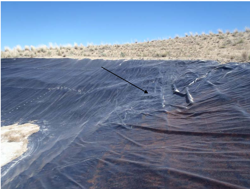
Xenon Upper Pit – Slope slumping under liner.
