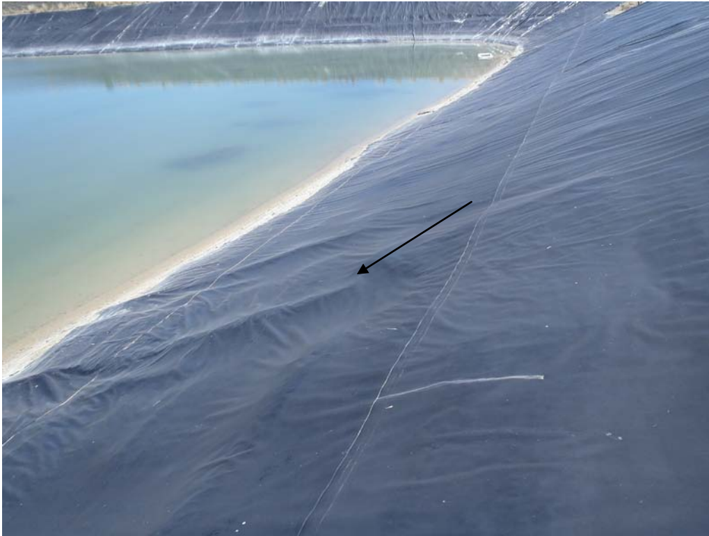
Xenon Upper Pit – Slope slumping under liner.
