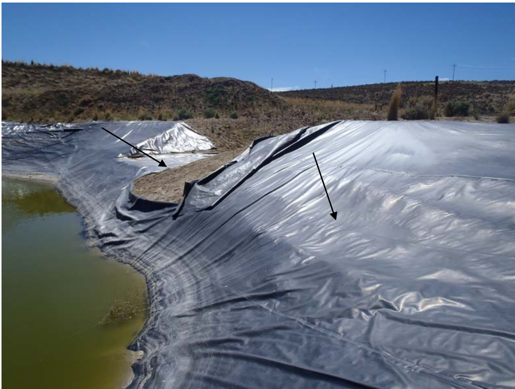
Xenon Lower Pit – Spillway liner tear and slumping.
