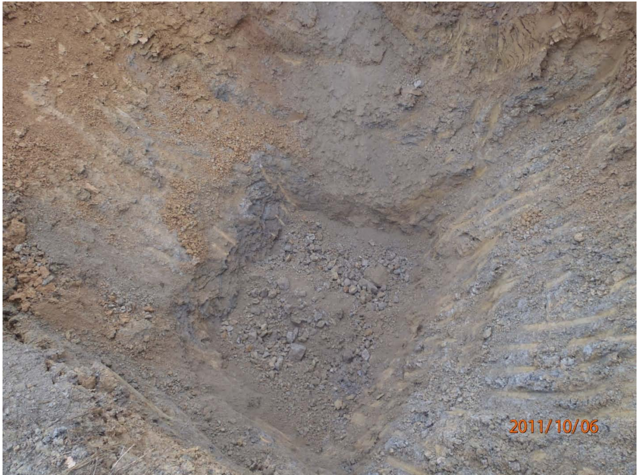
Visual representation of the remediated pit; depth presented is at 11 feet
