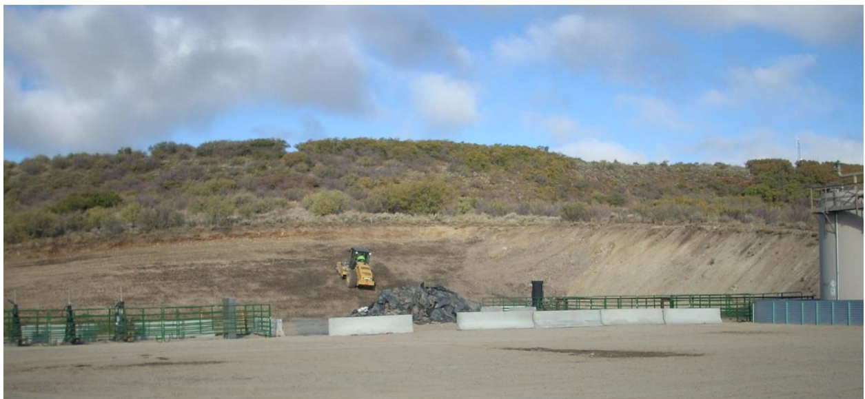
Photo 23: Pad 18C Compaction on the Cut Slope (10122010)
