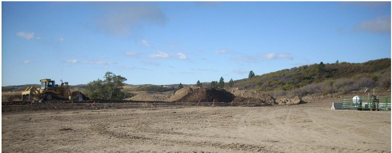
Photo 25: Topsoil Placement on Pad 18C (10122010)
