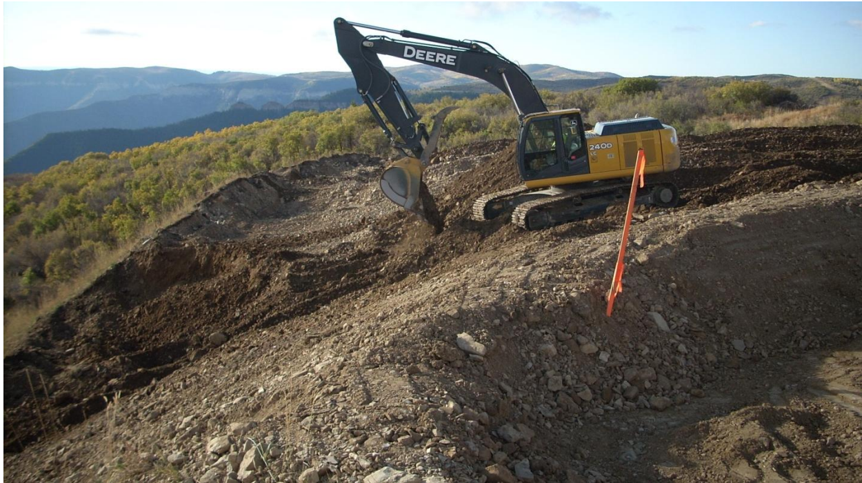
Photo 26: Working Towards Final Interim Fill Slope on Pad 18C (10122010)
