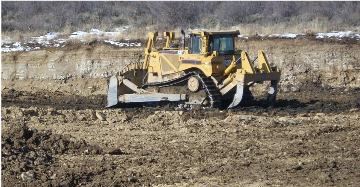
Photo 20: Pad 18A Placement of Amended Material and Fill Material Lifts (10292010)
