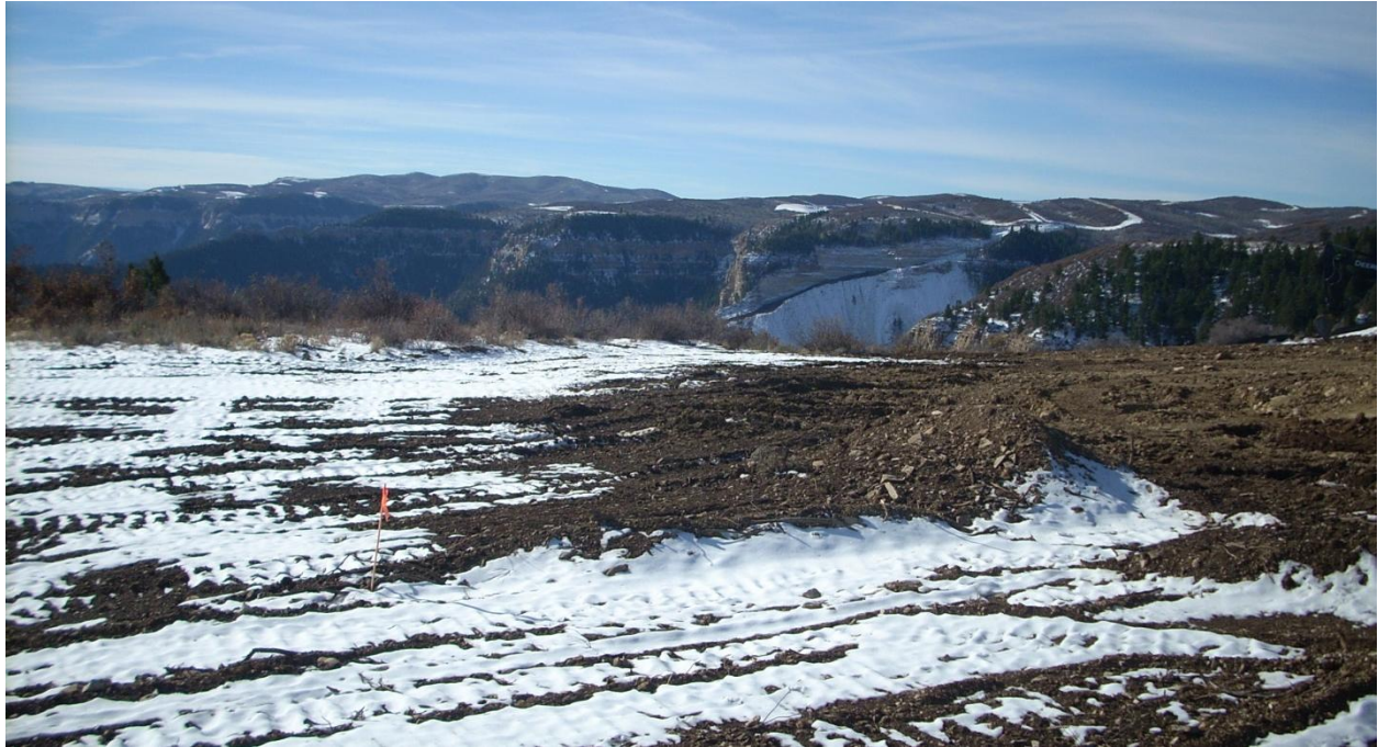
Photo 22: Rough Grade in Comparison to Final Grade and Topsoil Placement on Pad 18A (10292010)
