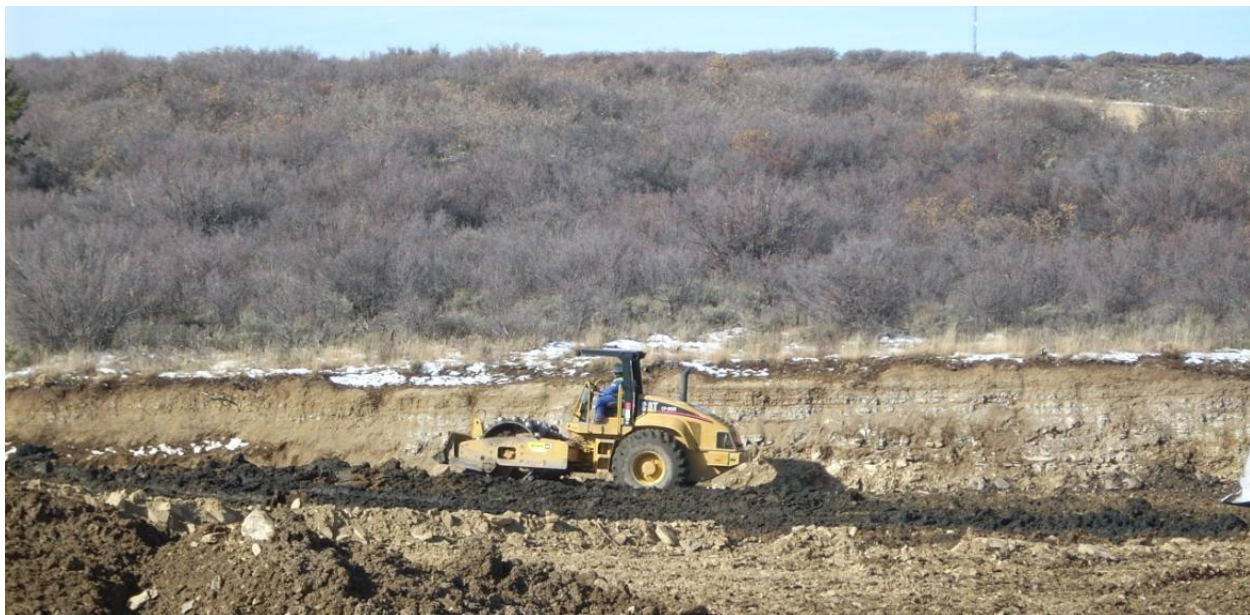
Photo 19: Achieving Appropriate Compaction of Backfilled Material (10292010)
