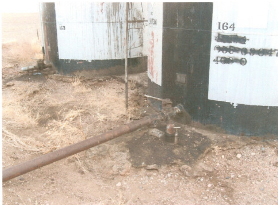
Oily soil at tank battery.
