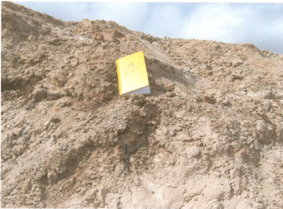
Small areas of localized oily soil remain in west wall of water pit excavation.
