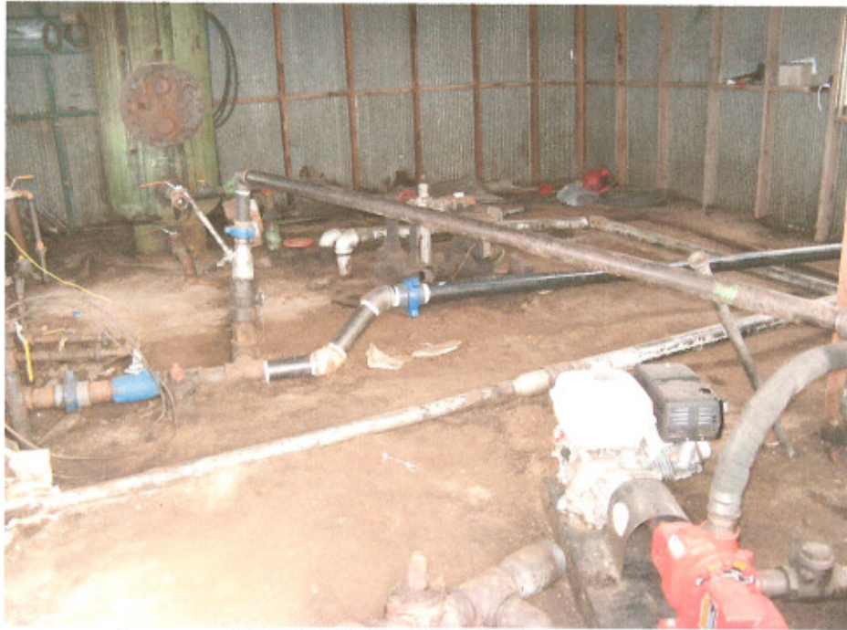
Oil saturated soils in treater shed.
