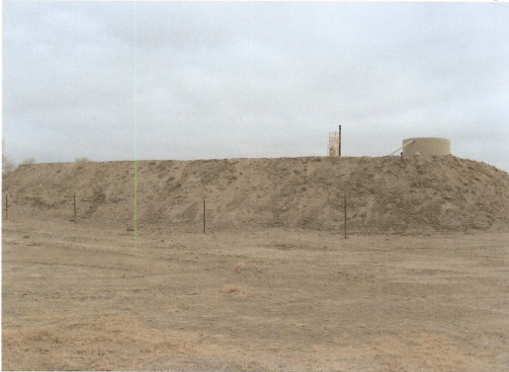
Disturbed area below water pit needs stormwater controls.
