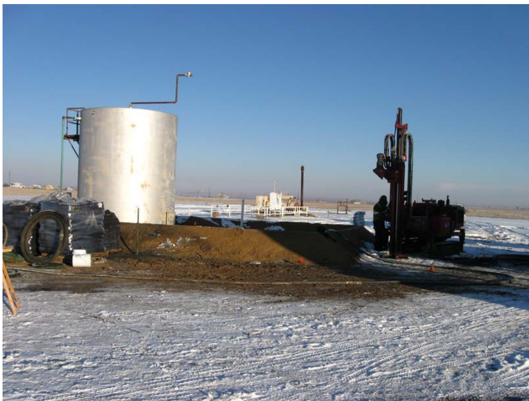
Photograph 4: Injection activities along the tank battery.
