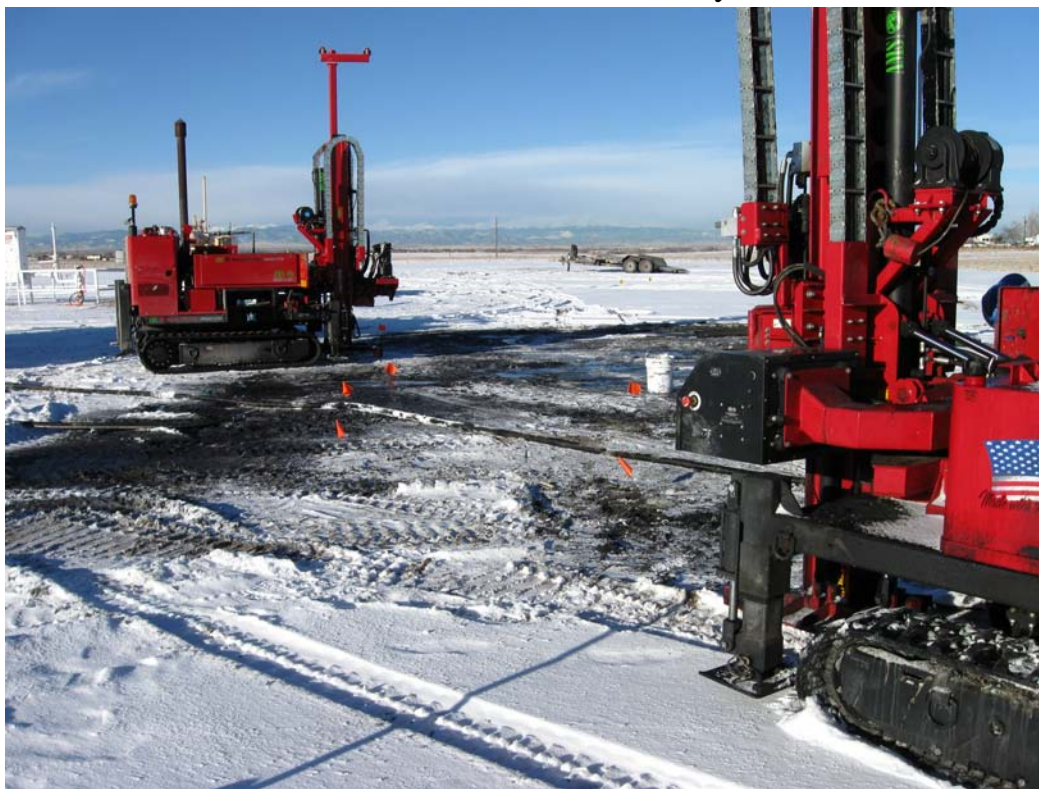
Photograph 3: Direct push rigs installing injection points.
