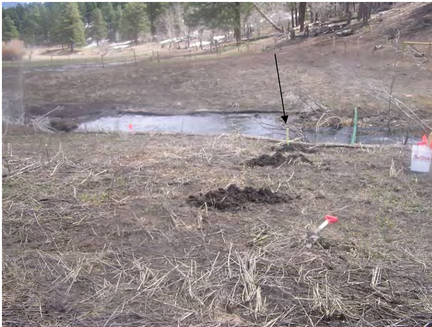
Photo 6: View of exploratory pits excavated perpendicular to creek. Arrow points to Pit 4; view is to the east. Pipeline across creek is visible in photo for reference. All pits encountered the impermeable liner at depths ranging from approximately 9 inches to 16 inches.
