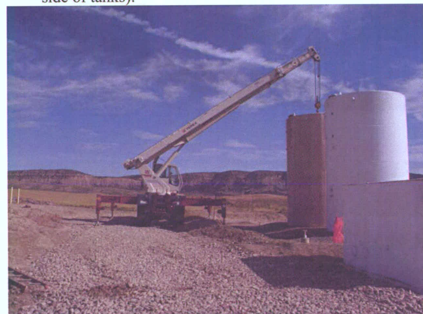
88. Preparing to remove north tank, Tank 3332.
