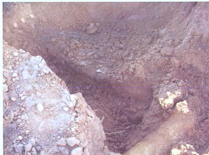
131. Excavation below east berm where free hydrocarbons were encountered.
