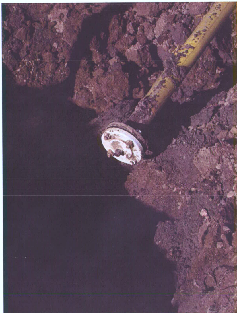
62. Capped sump inlet piping.
