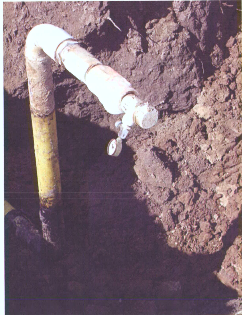
61. Capped sump outlet piping.
