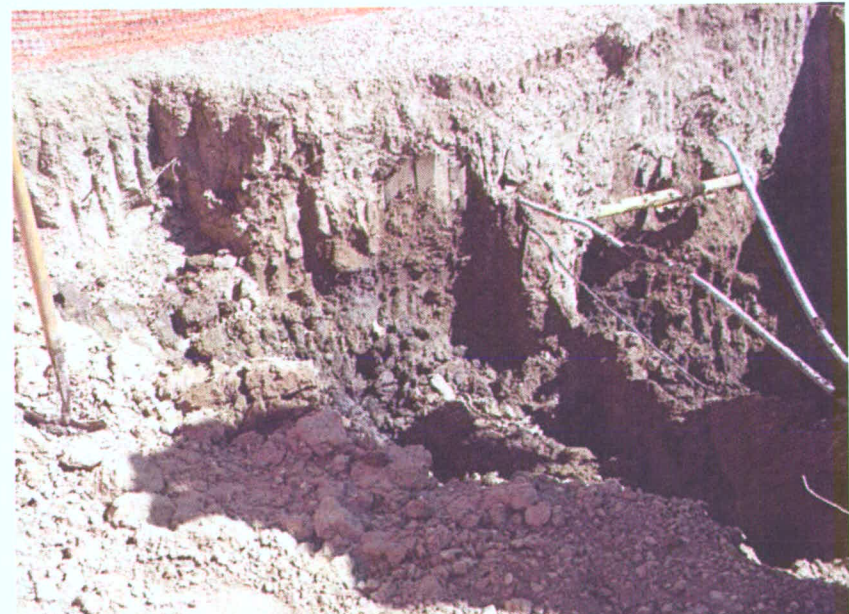
68. Contaminated soils near sump inlet piping.
