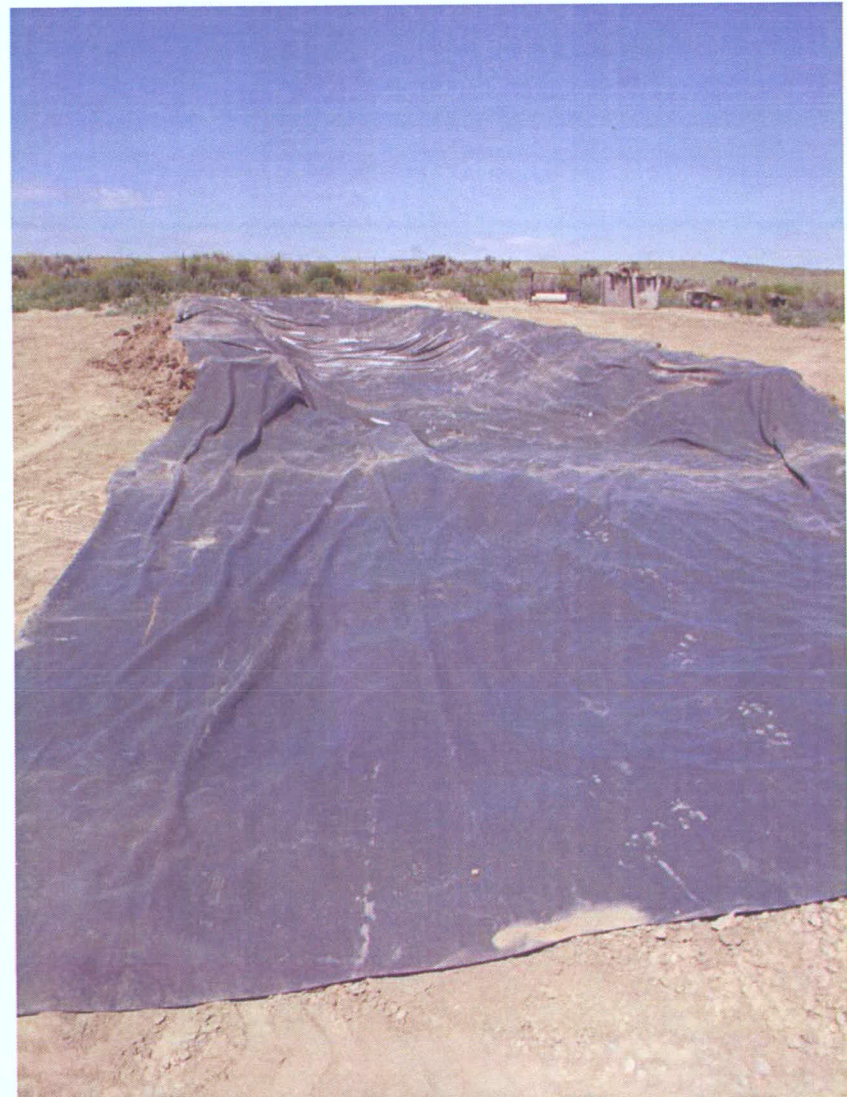
46. Contaminated soil stockpile liner prior to use.
