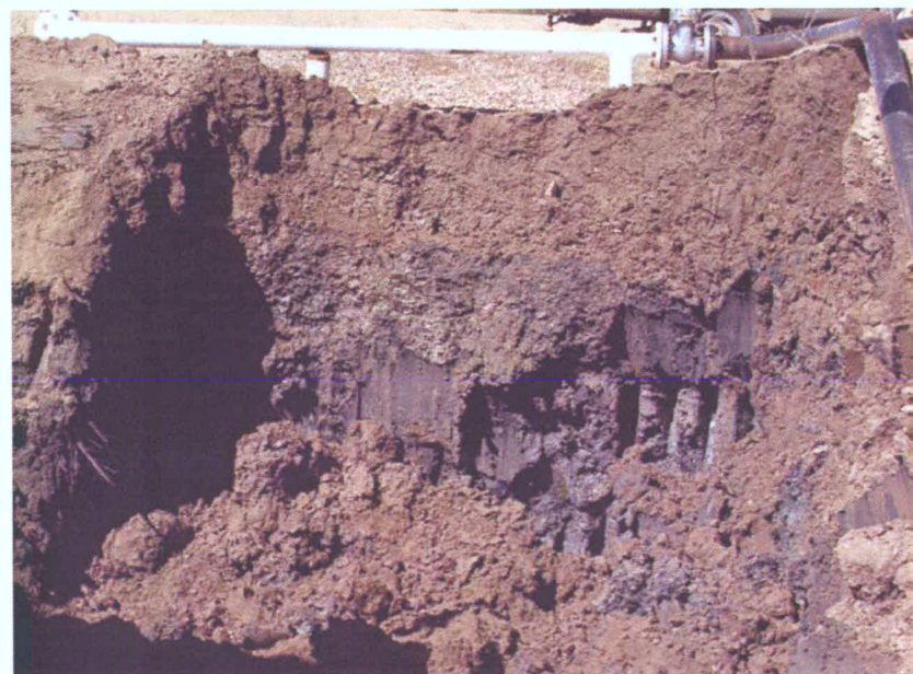
137. Excavation into bank below east berm near unloading line to tanks (voids near lower center).
