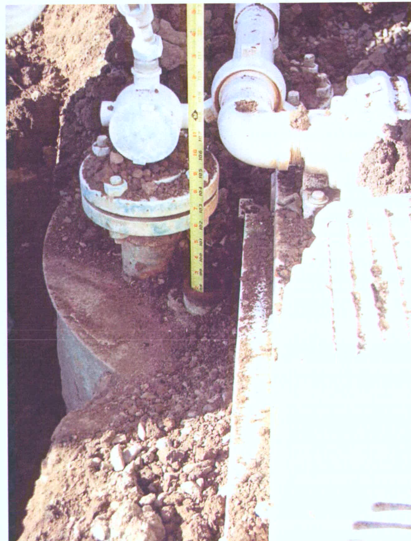
6. Measuring depth of sump.
