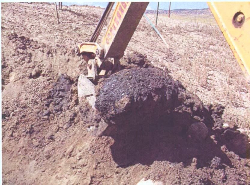
143. Oily gravels excavated from ditch on west side of truck unloading area.
