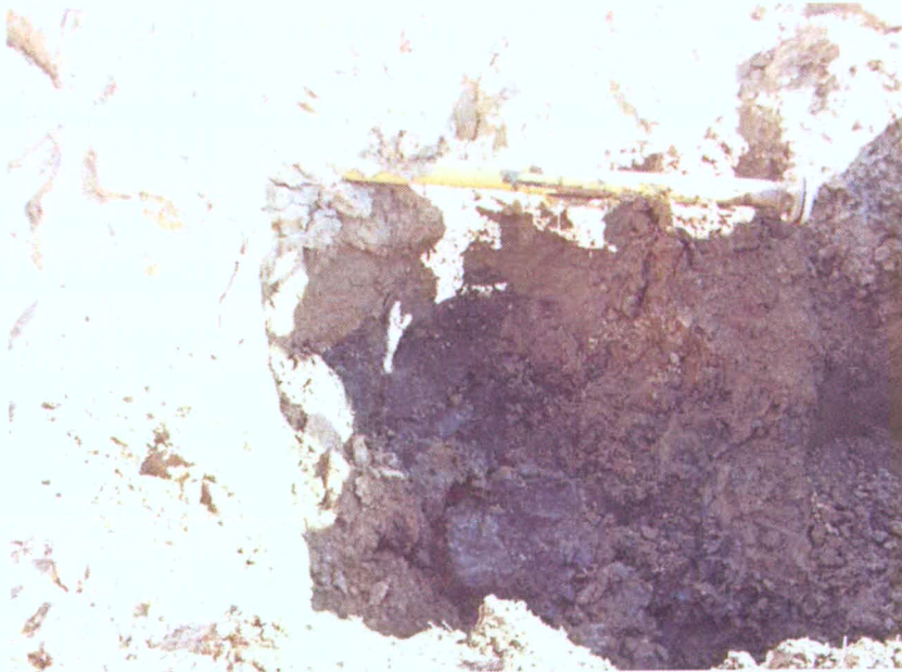
65. Contaminated soils beneath sump inlet on north side of excavation.
