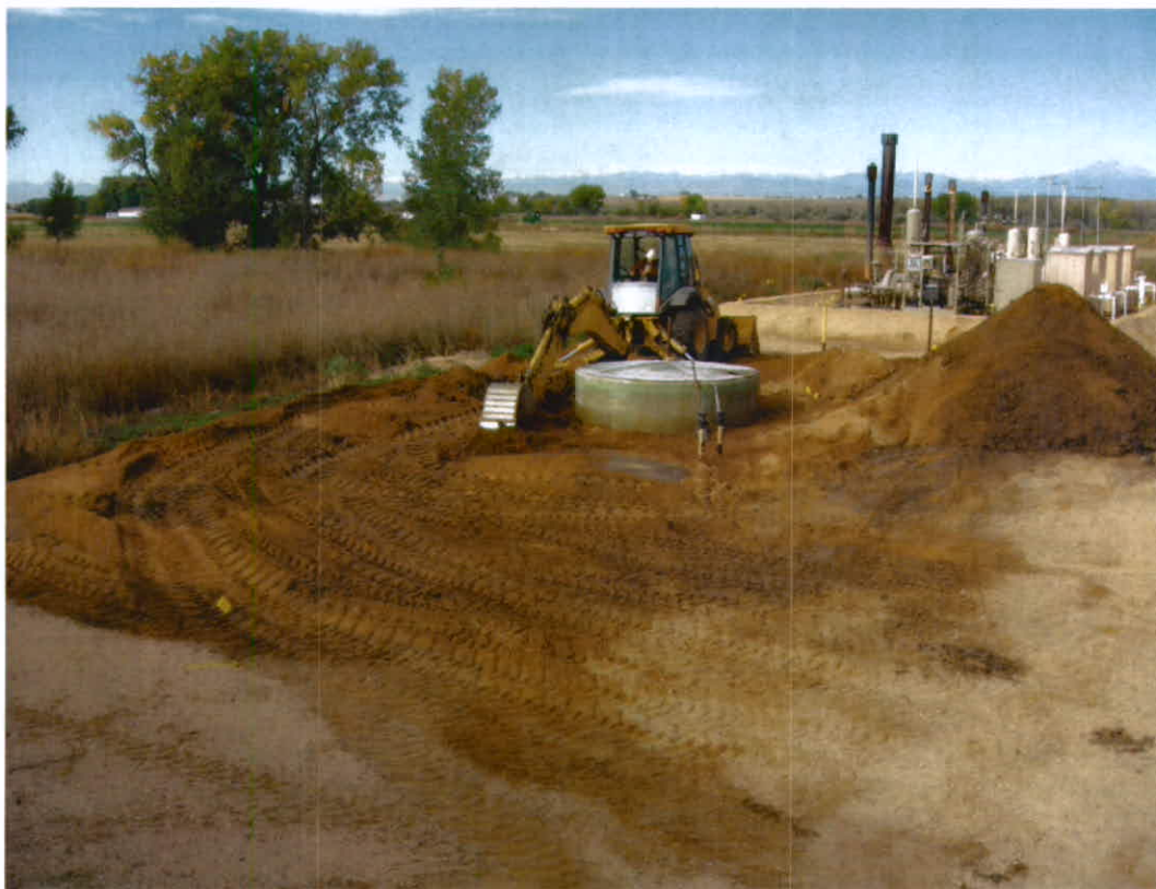
Photograph 2: Removal of tank battery soils. View southwest.
