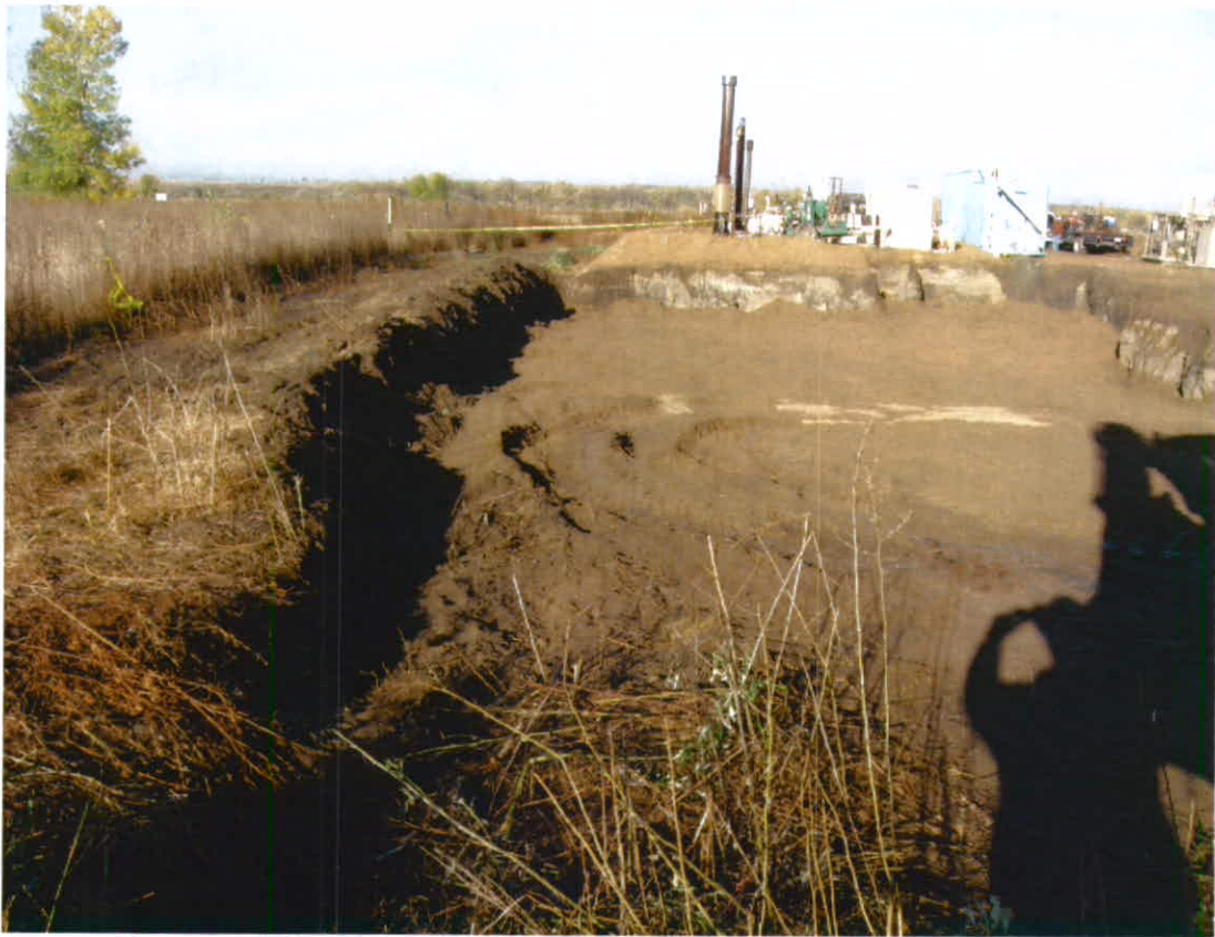
Photograph 3: Excavation partially filled with clean soil. View west.
