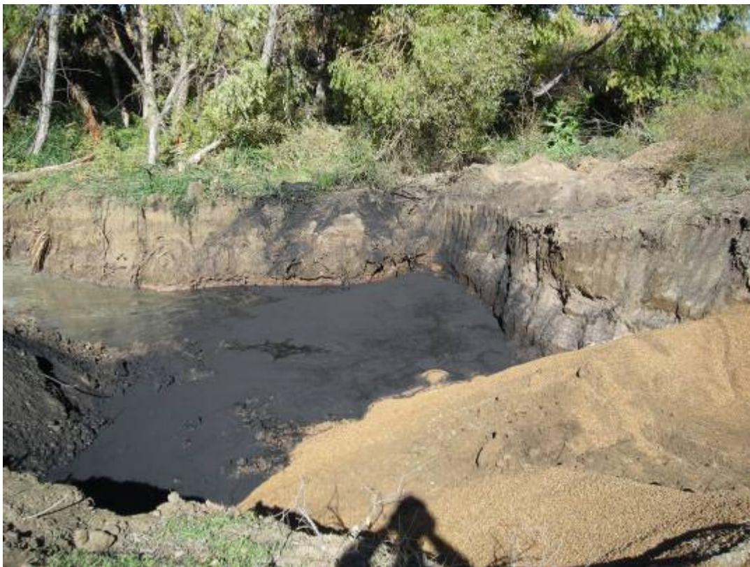
Photograph 2: Application of the groundwater amendment. View northwest.
