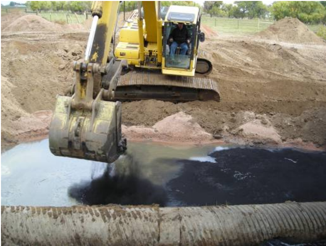
Photograph 5: Application of the groundwater amendment. View east.
