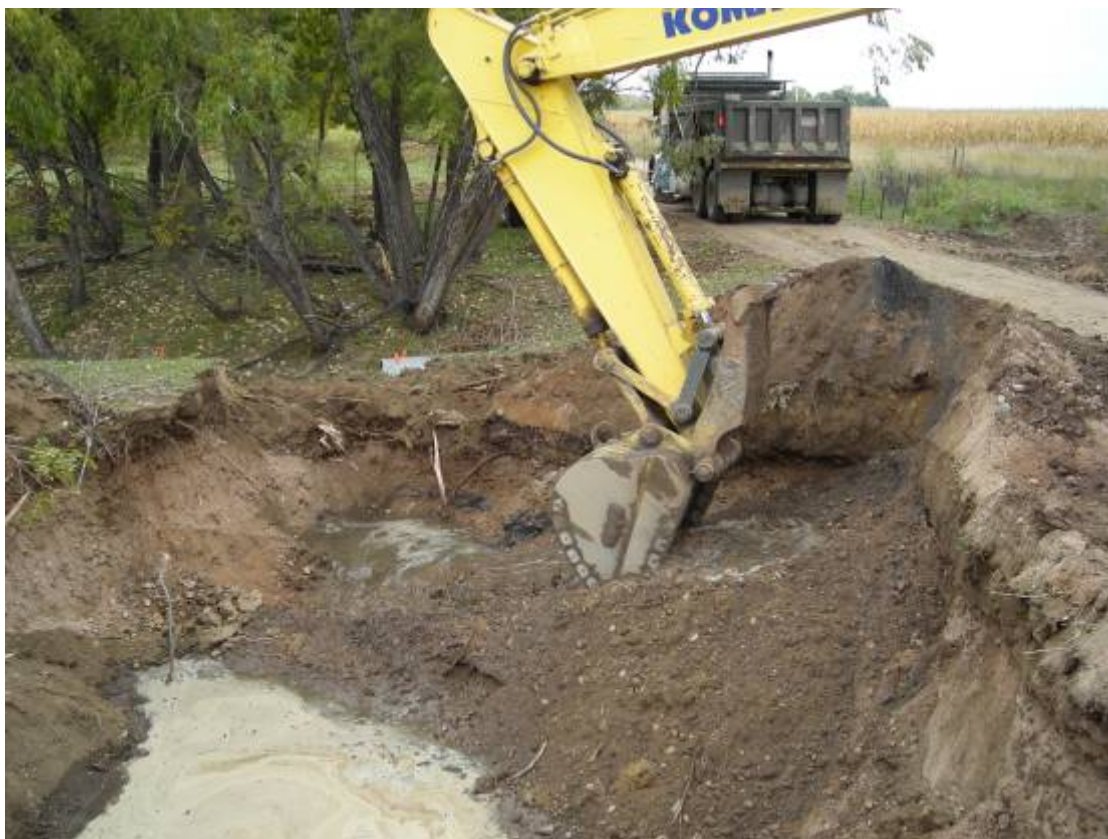
Photograph 3: Excavation of impacted soil south of the lease road. View west.
