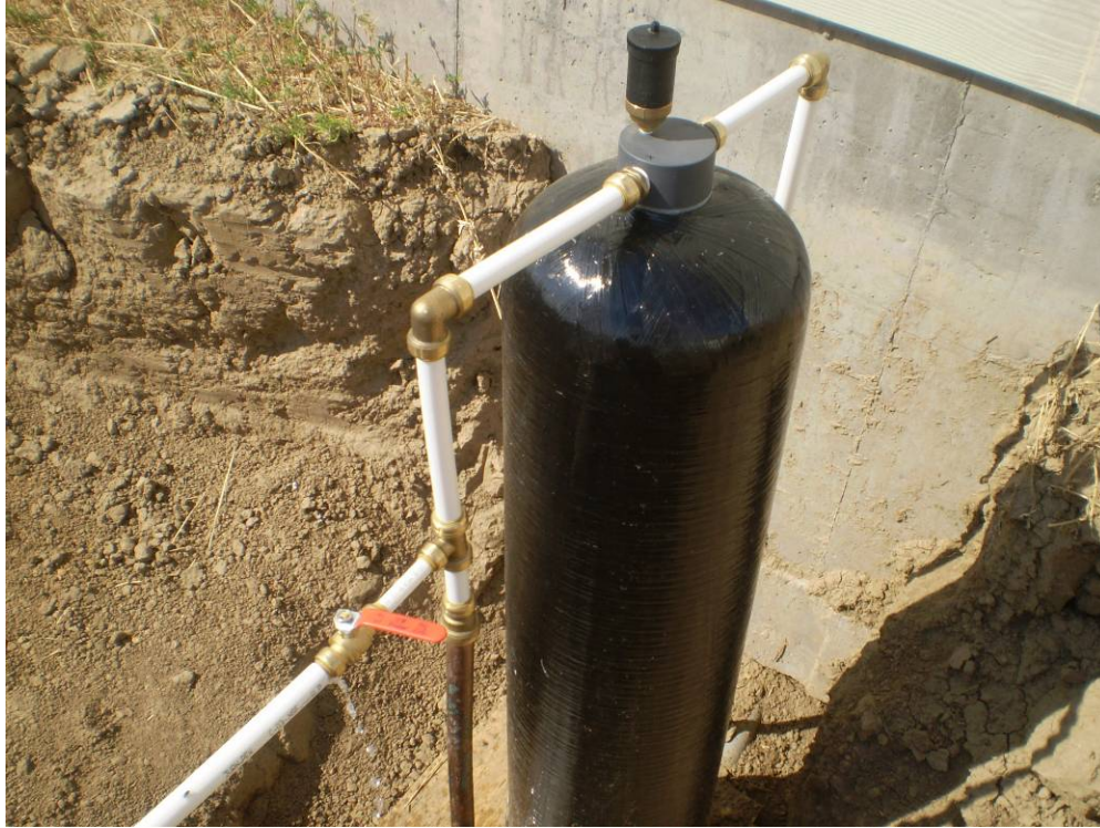
Photo #5 View of the pressure tank and the PVC by-pass
