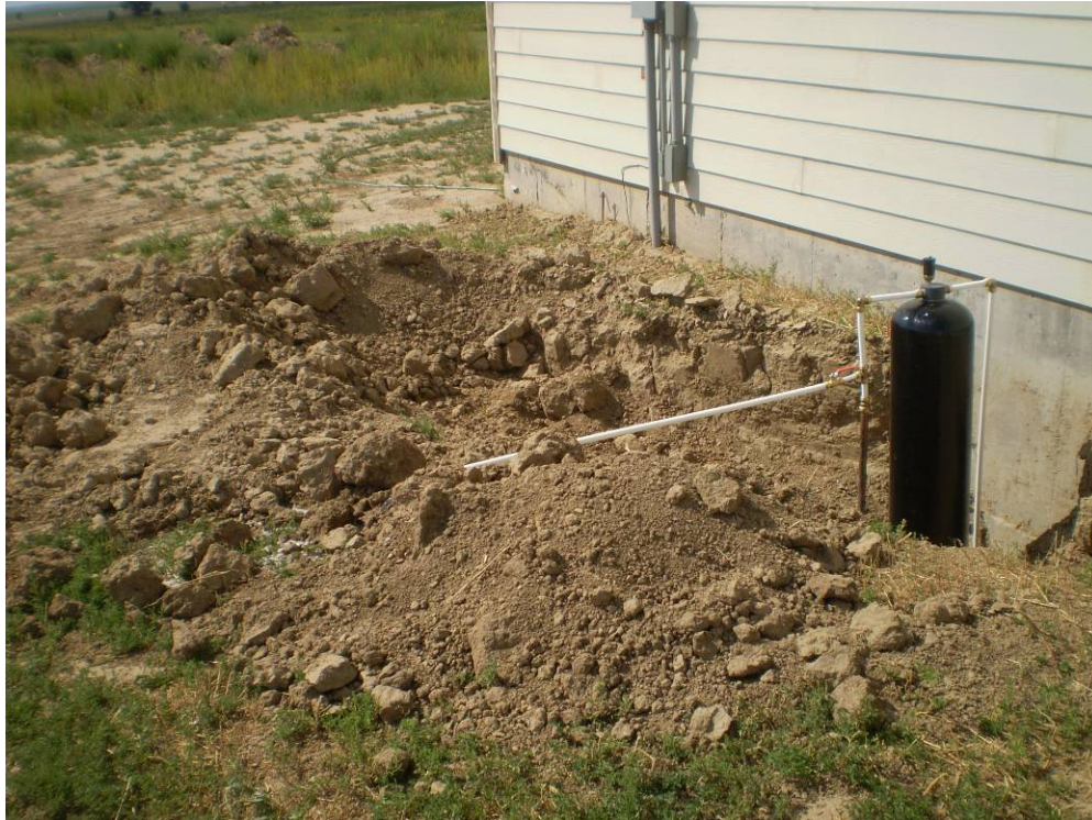
Photo #2 View of the PVC sampling extension and the pressure tank
