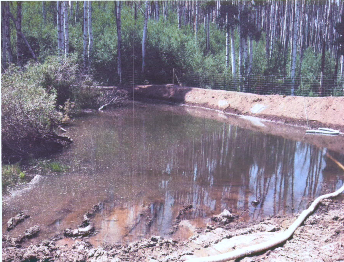
Photo 1- Lined and bermed impoundment at the point source of Rock Spring
