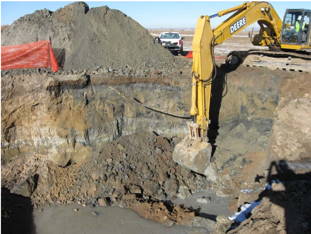
Photograph 2: Excavation of impacted soils in northeastern corner. View is north.
