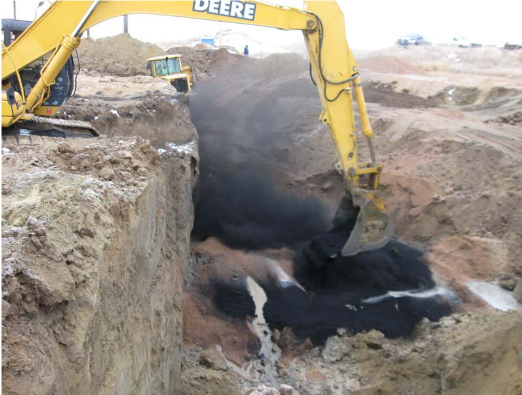
Photograph 3: Installation of carbon remediation product to the base of the excavation. View is southwest.
