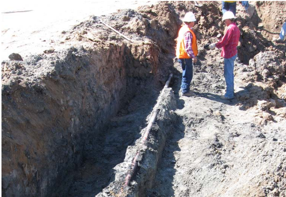
Photograph 2: Hand location and excavation of impacted soils along DCP sales line.
