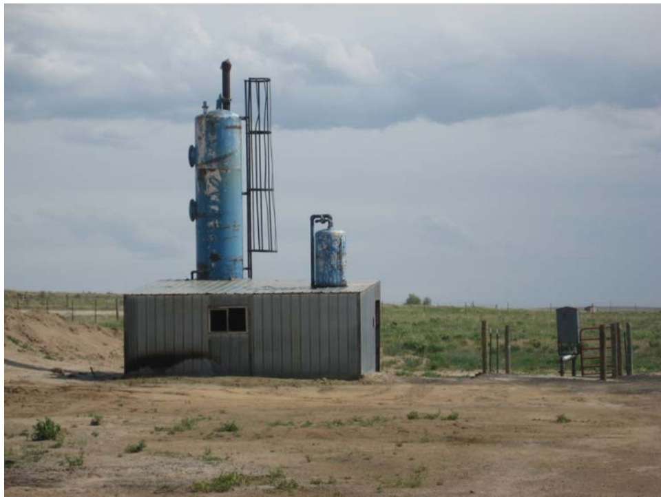
Photo 2. Separator on battery site for Myers 32-3 2
