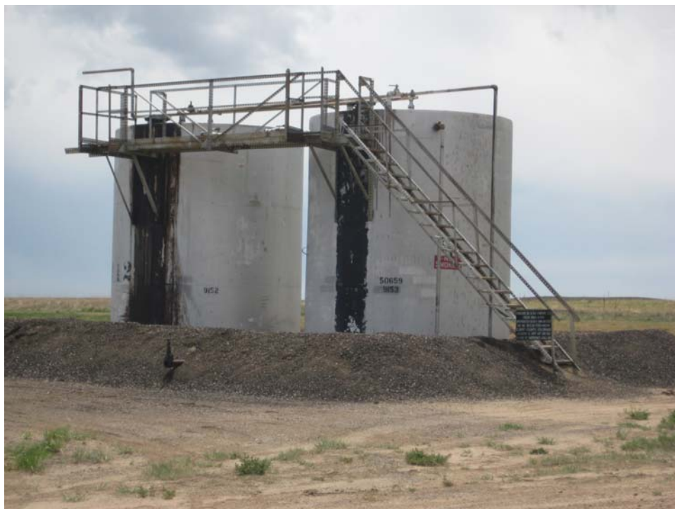
Photo 2. Two 300 BBL tanks used for water and production
