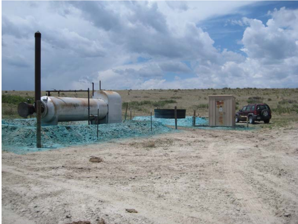
Photo 3. Looking southwest at buried fiberglass tank and horizontal separator
