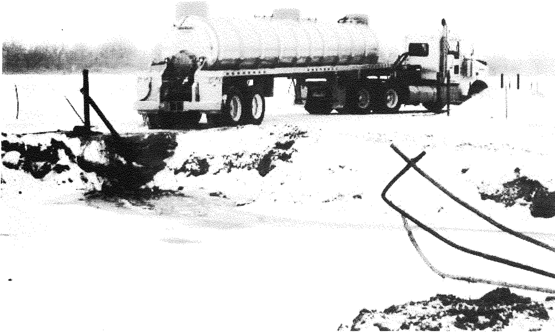
Photo 3 - A vacuum tanker truck removes ground water from the cleanup excavation.
