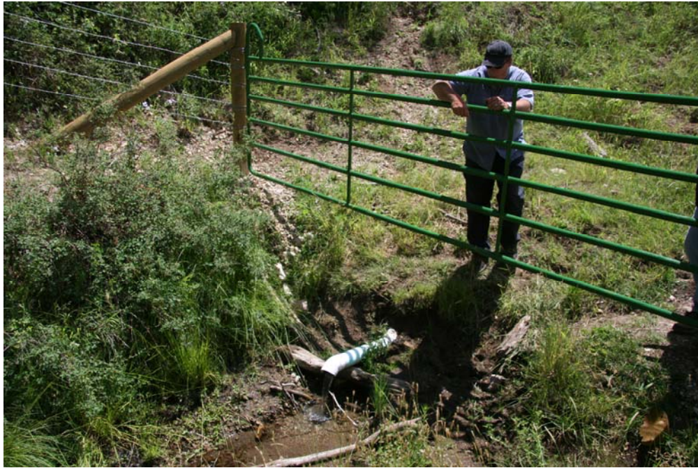
Figure 3 – View to East Below Discharge Pipe. Orange Flagging in Creek Marks Location of Cistern Outlet Pipe. Cistern Vent Pipe (1-inch diameter PVC) is Tied to Steel Fence Post Shown in Background of Photograph
