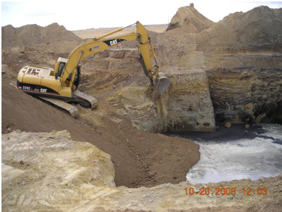
Photograph 4: Backfilling the northern excavation.
