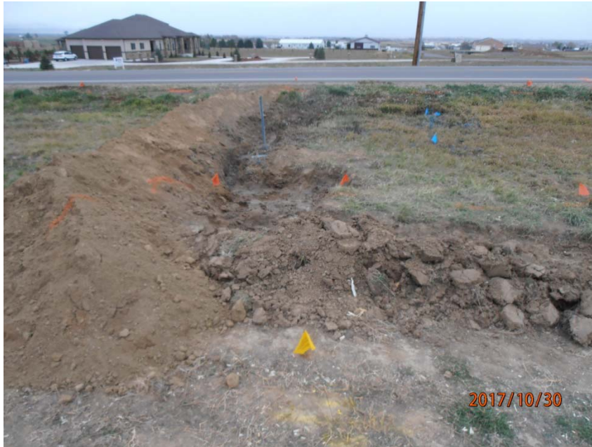
Photo 1: View at terminal location of released liquid migration in ditch along Highway 60. Berm built in ditch on dowgradient, west end of release. Photo views to North.
