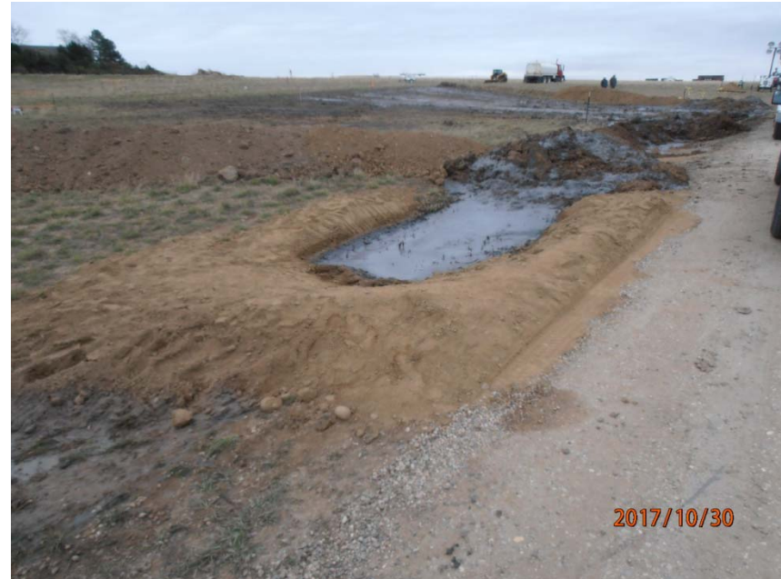
Photo 4: View at release location where liquids migrated into ditch along driveway. Berm constructed in driveway ditch to contain release liquid. Photo is viewing southeast.
